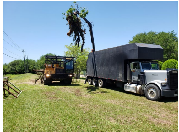
Debris removal from Oyster Creek
