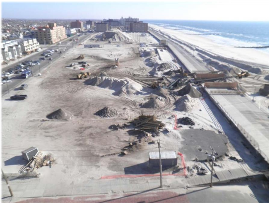
Sand Reclamation and Screening Site
