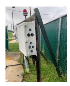
Further evidence of the corrosiveness H2S can be seen on the main disconnect and meter can that compromises a weather-tight seal crucial for safe operations.
