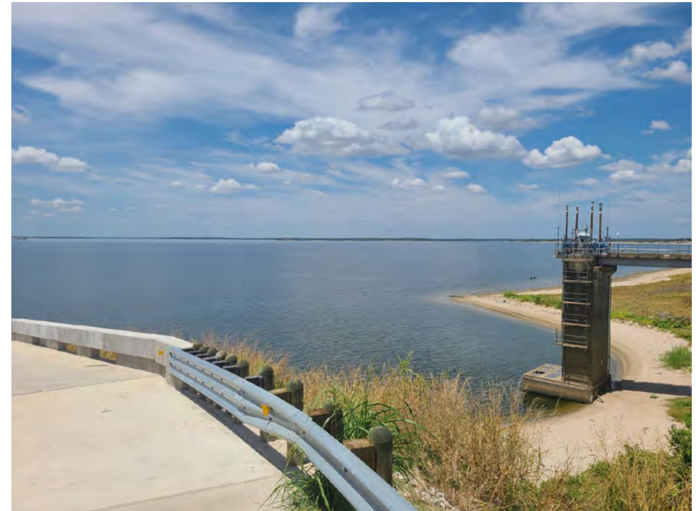
Lake Somerville Intake Facility
