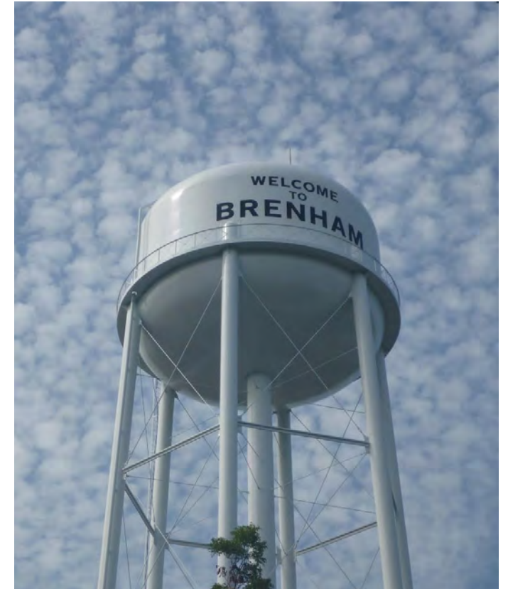
Church Street Elevated Storage Tank
