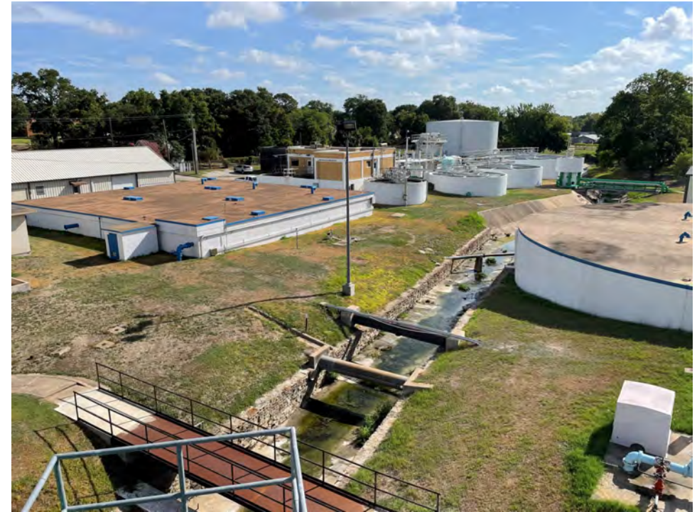
Surface Water Treatment Plant
