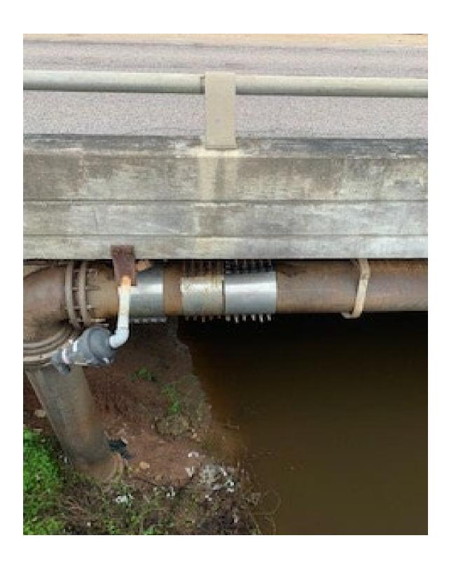
Deformed clamps around piping showing loss of structural integrity of piping which has been accelerated by the tightening of compression bolts on the clamp.
