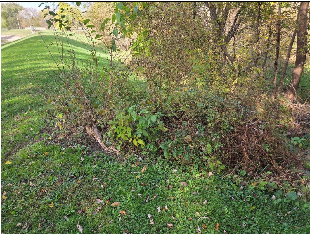
Photograph: 24 Church Street Diversion photo, viewing in the westerly direction. Vegetation to be removed.
