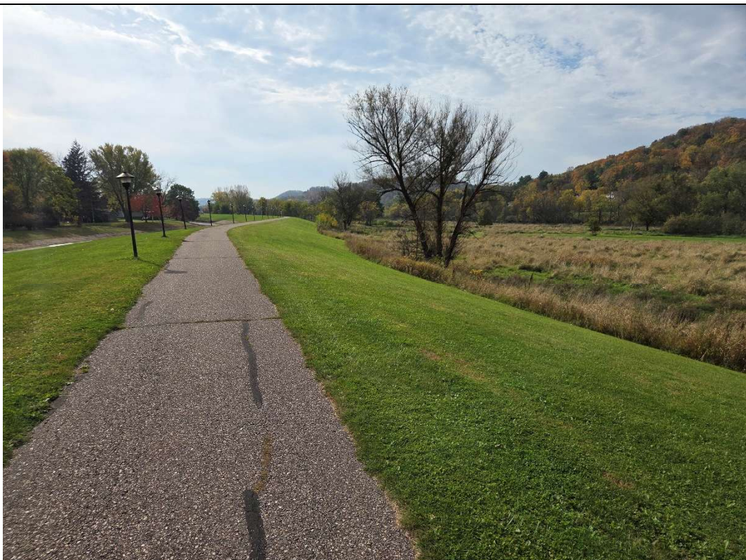
Photograph: 30 | Upper main dike photo south of STH 14, viewing southerly.
