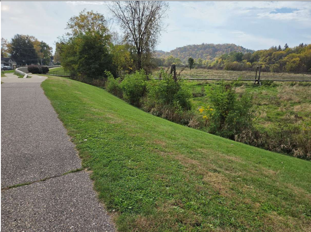
Photograph: 31 Upper main dike photo, viewing southerly toward existing bridge. Trees and brush to be removed at toe of levee.
