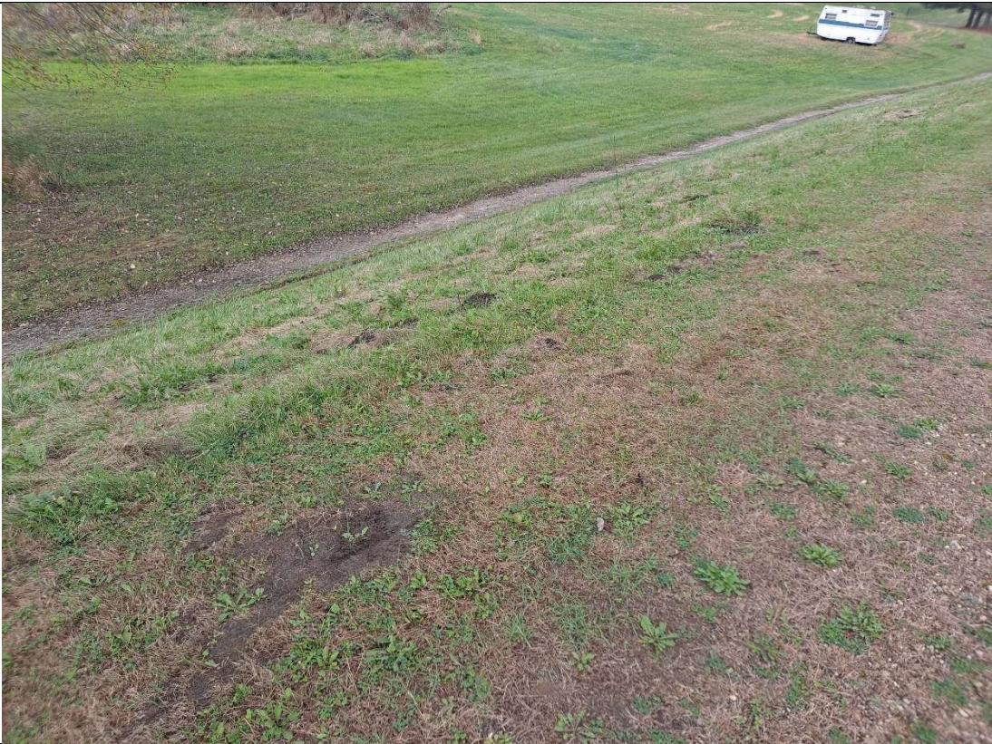
Photograph: 3 | Allison Park dike photo, viewing in southwest direction.
