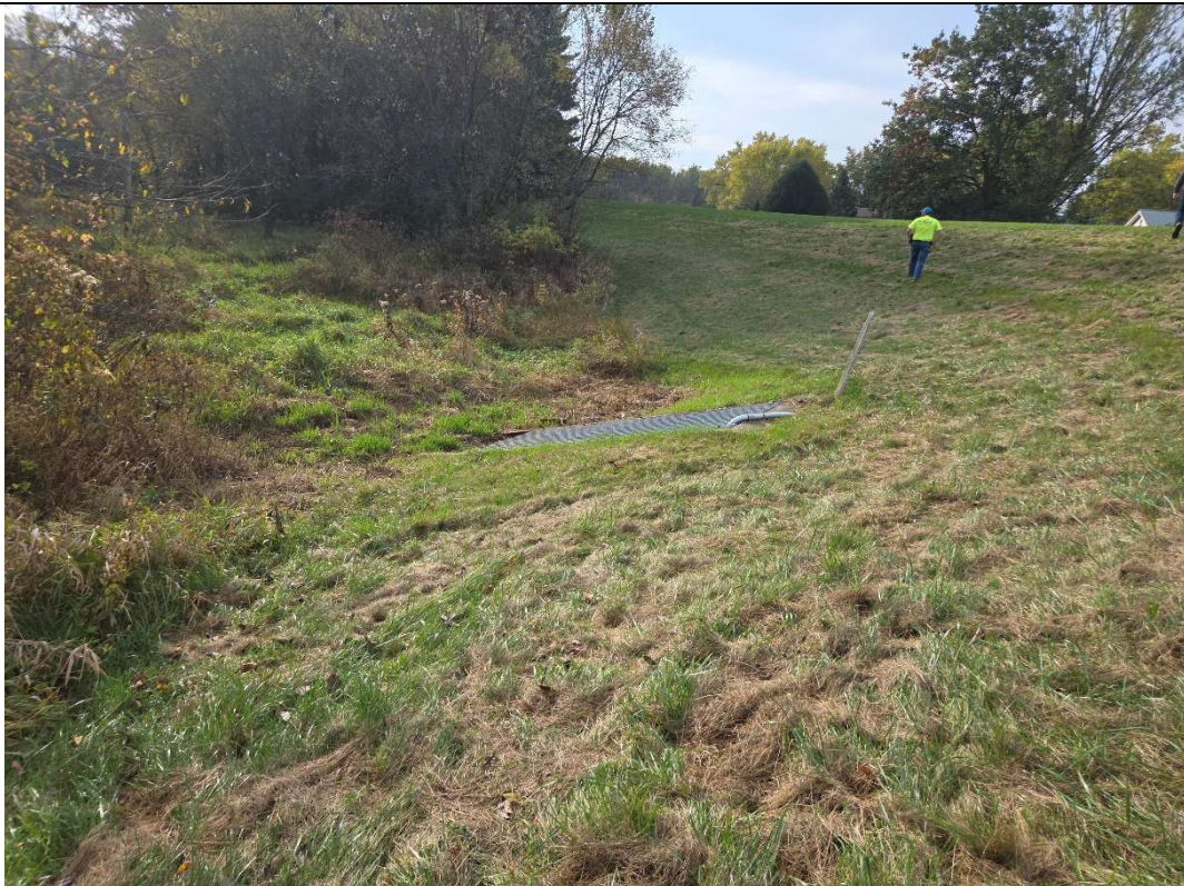
Photograph: 4 | Inlet and Valve at approximately Station 26+50.
