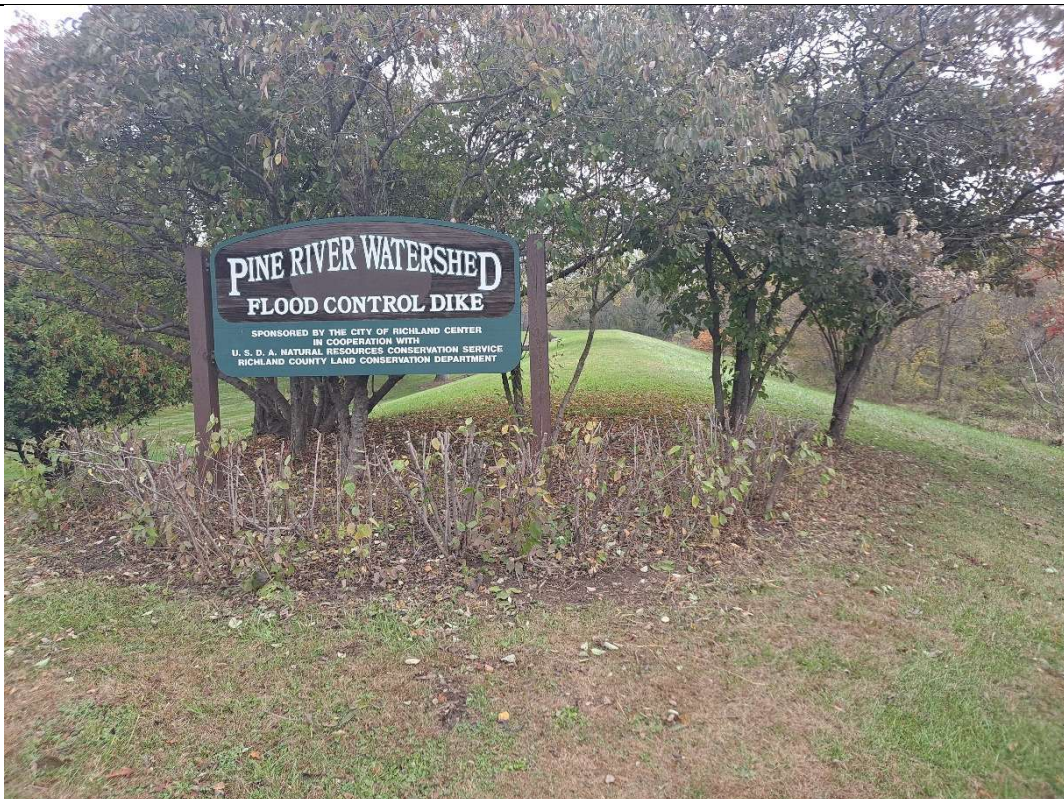
Photograph: 19 Taken from STH 80 viewing sign to the northeast. Trees and shrubs to be removed at base. Roots to be left in place and treated.
