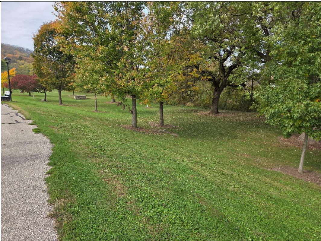
Photograph: 29 | Photo of dike Northeast of STH 14 viewing Southwest.
