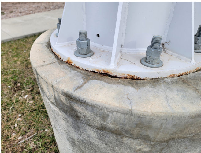
5. CORROSION ON BASE OF SLIDE SUPPORT
