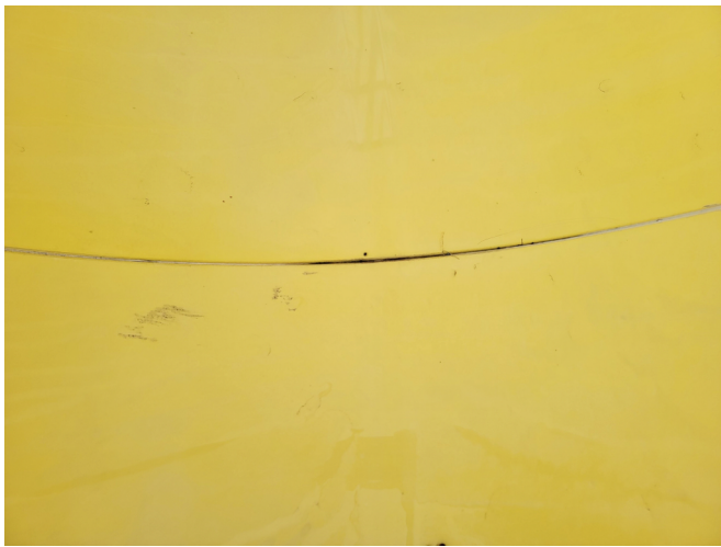
3. MISSING SEALANT
