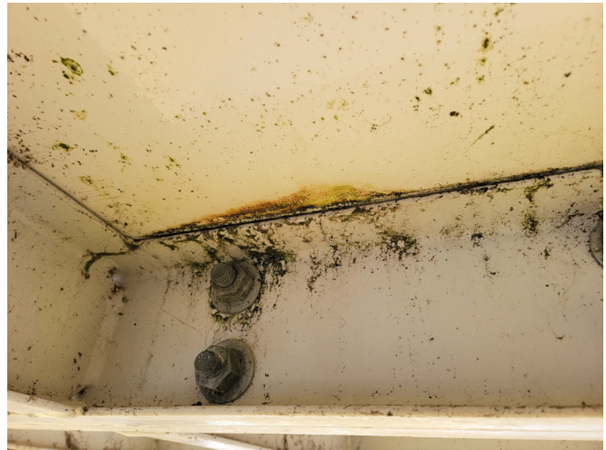
6. DIRT/ALGAE AND CORROSION UNDER PLATFORM
