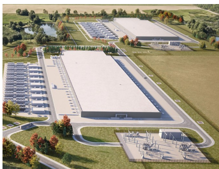
This artist rendering shows the 700,000-square-foot data center facility currently under construction on 570 acres, visible from U.S. Highway 151, in Beaver Dam (from Meta news release)
