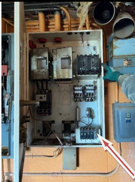
Photograph D-1: Mini-Storage Bldg, pump Rm: Sample 1A black 'Bakelite' electrical switches (about 7 large and 5 small) 30% chrysotile asbestos-containing material (ACM), Category II, non-friable, intact. Orange wall paint contains lead (all paint contains lead).
