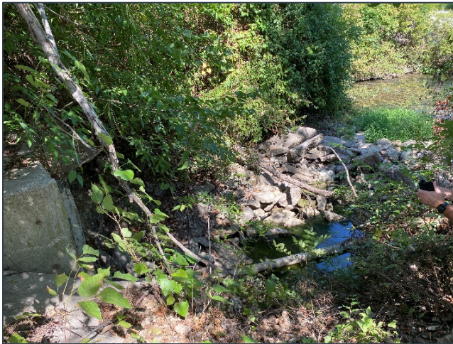
Picture 17. View east downstream from crest
