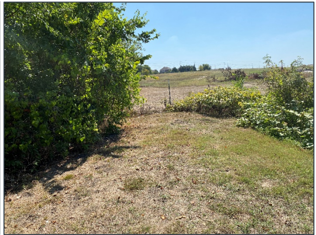
Picture 2: Crest of embankment looking south
