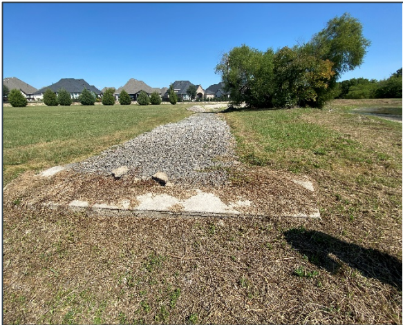
Picture 7. End of upstream embankment
