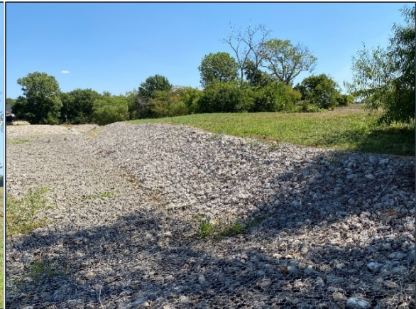
Picture 10. Gabion spillway north of embankment
