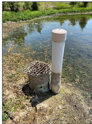
Picture 16. 16" PVC inlet structure
