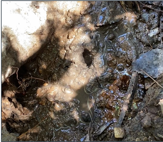
Picture 13. Seepage observation
