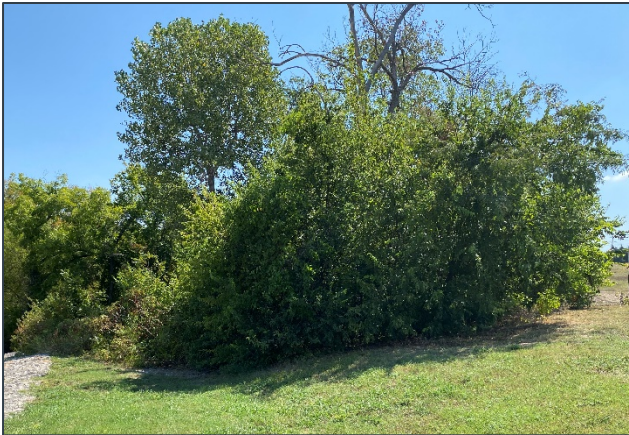
Picture 9. Vegetation east side of embankment
