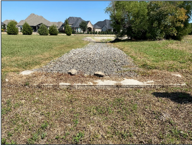
Picture 21. Service spillway view looking downstream
