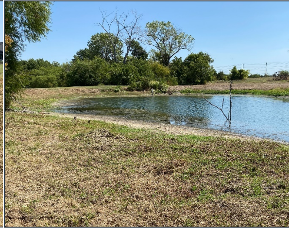
Picture 6. Upstream embankment looking south
