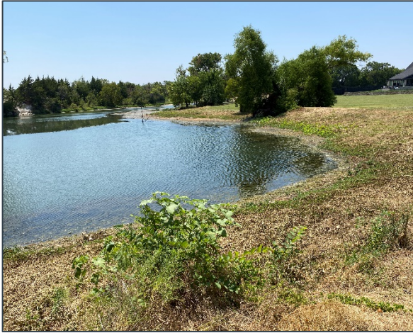
Picture 5. Upstream embankment looking north
