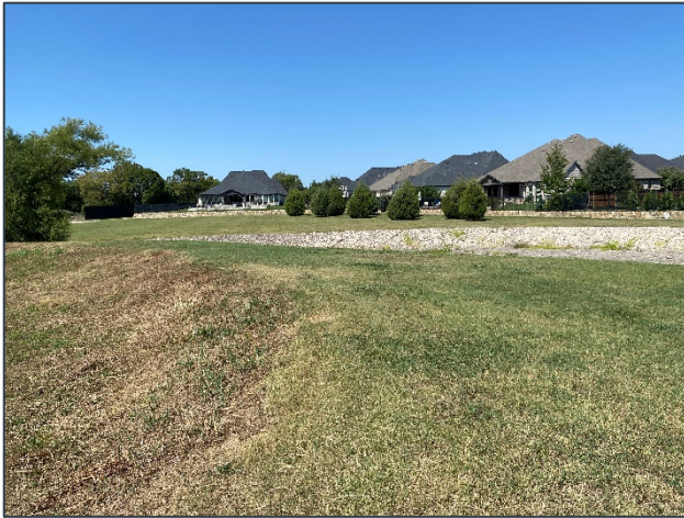
Picture 1: Crest of embankment looking north
