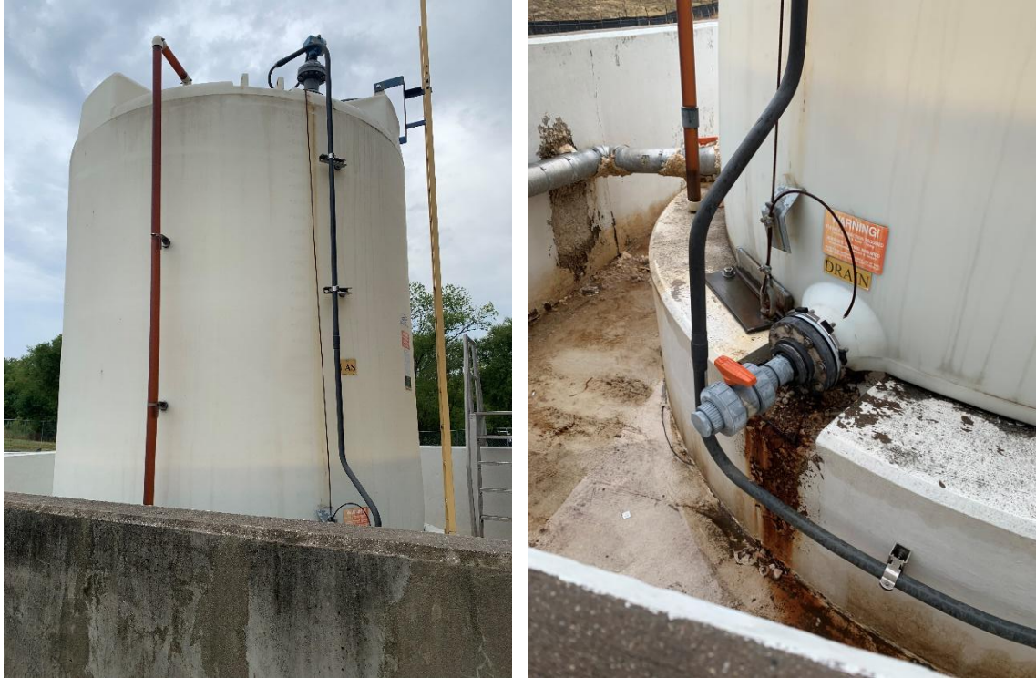
Figure 2-3: Bulk LAS Tank and Containment Area
