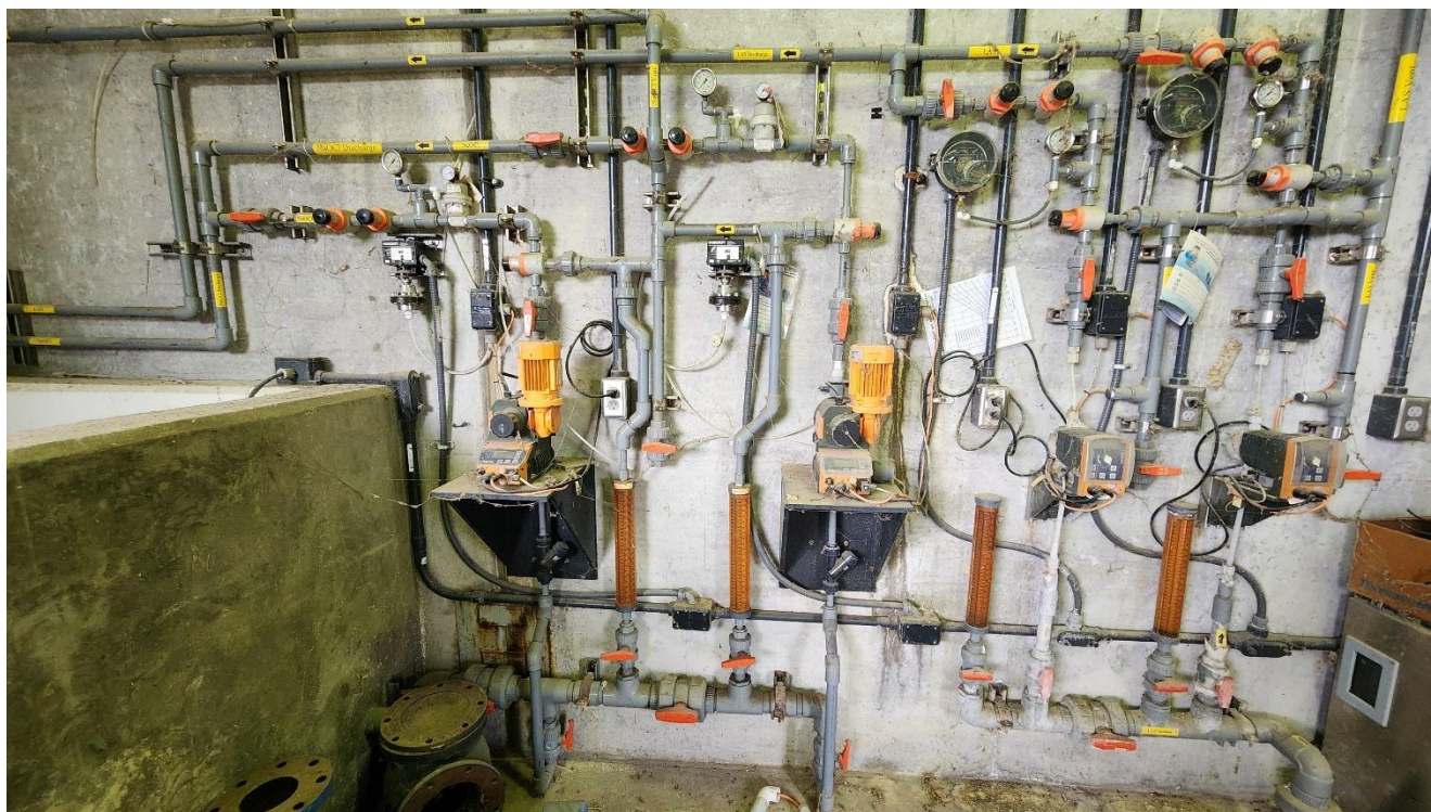
Figure 2-4: Sodium Hypochlorite and LAS Metering Pumps
