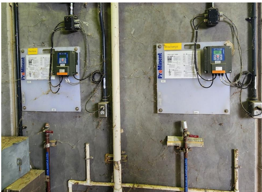
Figure 2-5: Chlorine Analyzer Controllers
