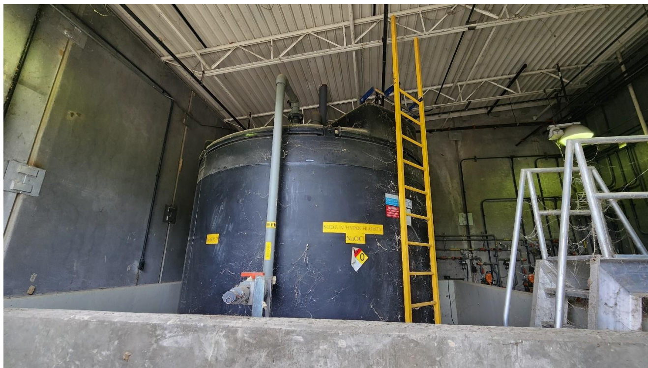
Figure 2-1: Bulk Sodium Hypochlorite Tank
