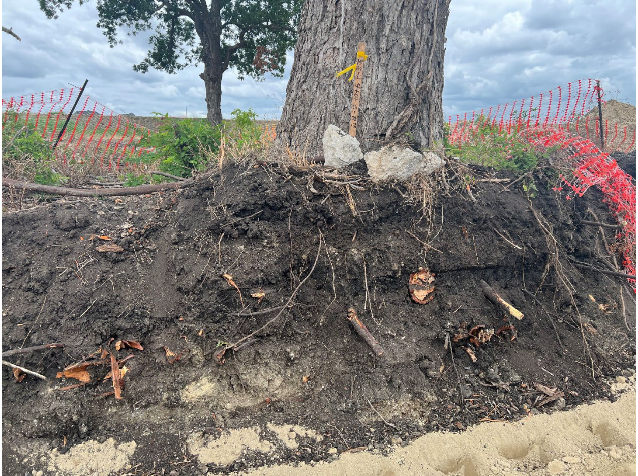
Tree 144 – significant root damage from road grade cut. Tree 146 (another pecan tree) in background demonstrates dense foliage in canopy by comparison.
