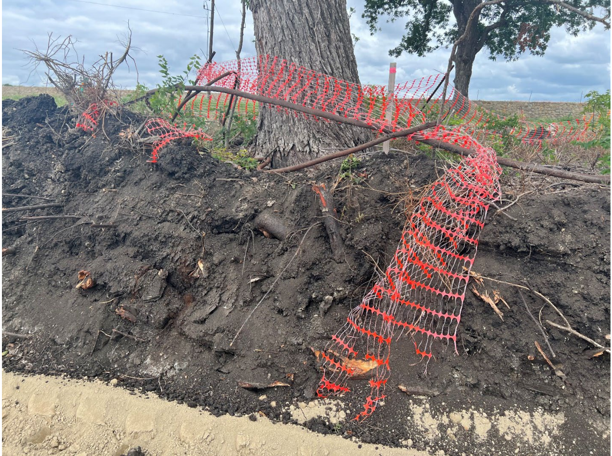
Tree 145 – significant root damage from road grade cut.
