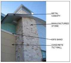
that are at least nine (9) feet above grade on non-residential buildings and on the third floor and above for multifamily buildings. Textured and painted concrete tilt wall shall be limited to 50% on the front façade and 75% on the side façades. Windows, doors, porches, gables, balconies and accent materials shall be excluded from the façade area for the purposes of calculating primary building materials.
