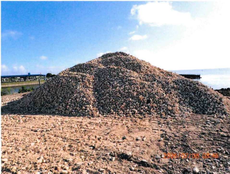
Figure 5. Bedding stone stockpiled at Borrow Site A.
