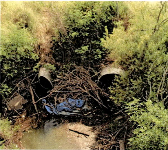
Photograph of upstream side this summer after a rain Note the collapsed end of the pipe on the left.
