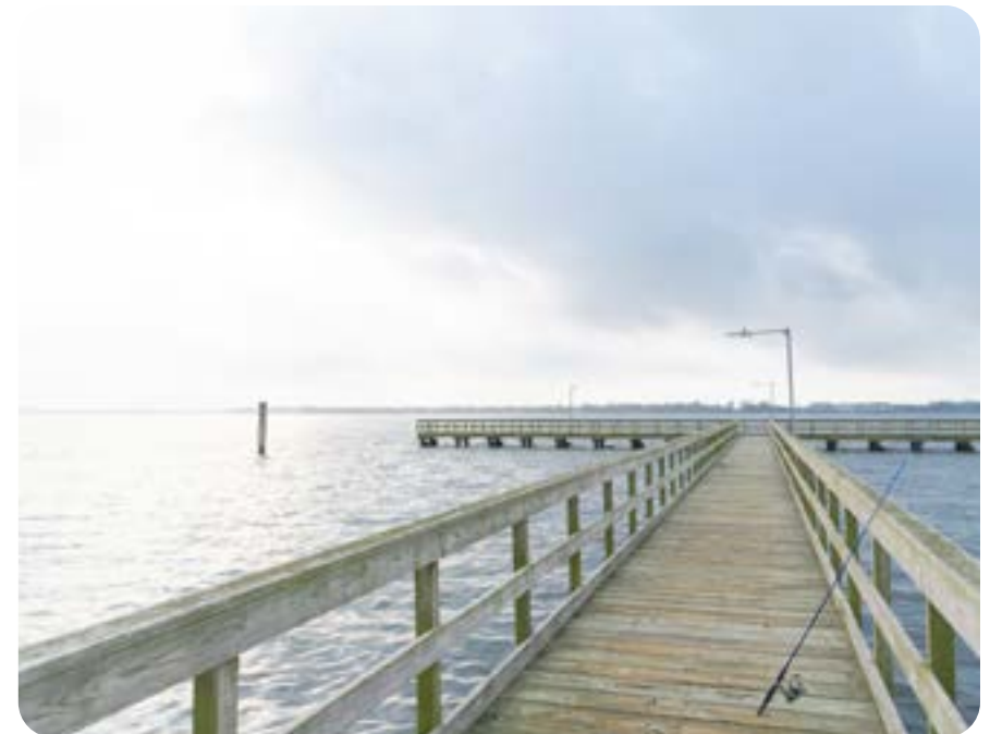
Port Lavaca Boardwalk
