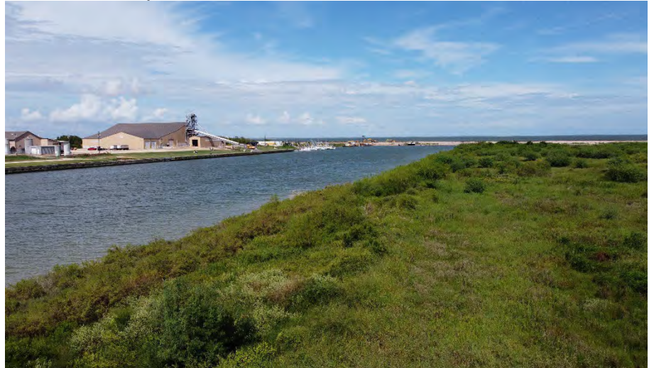
Figure 8: Aerial view to the East. Tidal marsh fringe is visible at the base of a berm contains a relict disposal area.
