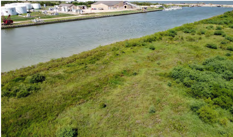
Figure 3: Aerial view of the Northern end of the project area looking East towards Lavaca Bay. Confining berm is visible separating wetland A from adjacent disposal area.
