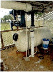
Photo 6 – Description: Light Pic 1
