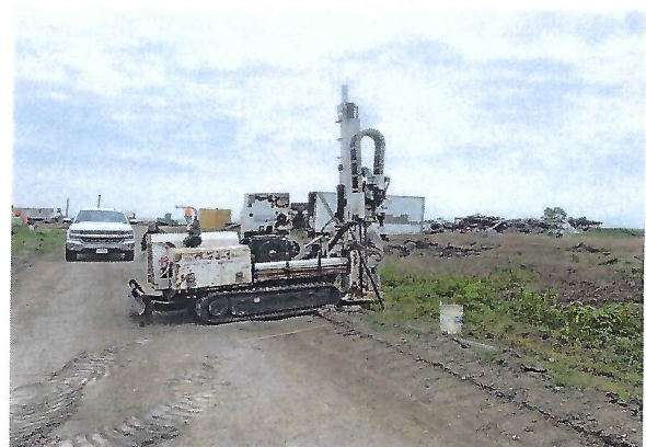
No. 8 View of SB-4 location at the west side of the site.
