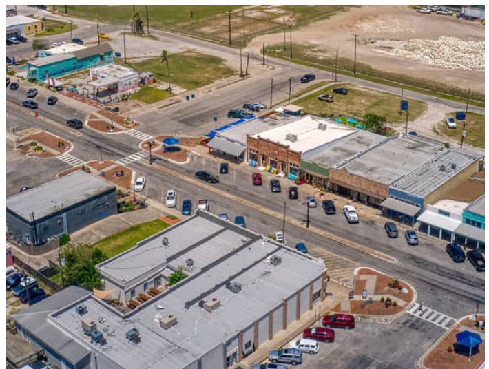
Rockport, Texas, Heritage District at South Austin Street, bulb-outs and streetscape Source: Visit Corpus Christi
