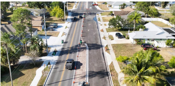
Port Saint Lucie, Florida, coastal roadway reconstruction with pathways and medians Source: City of Port Saint Lucie
