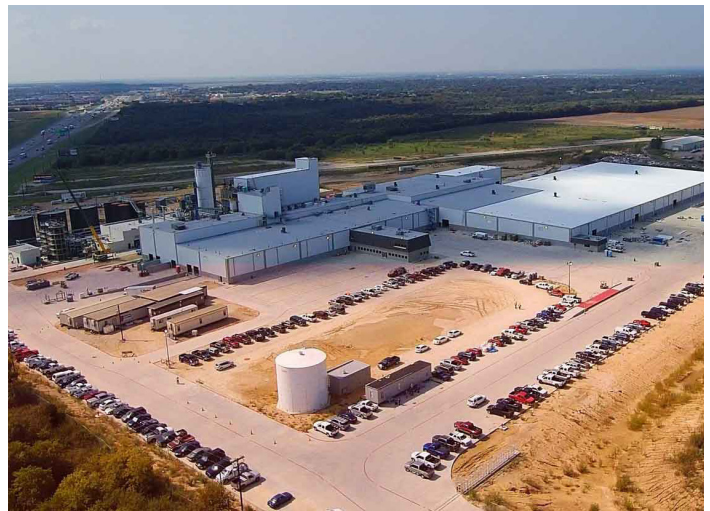
Asphalt processing plant Source: Cummings Electrical
