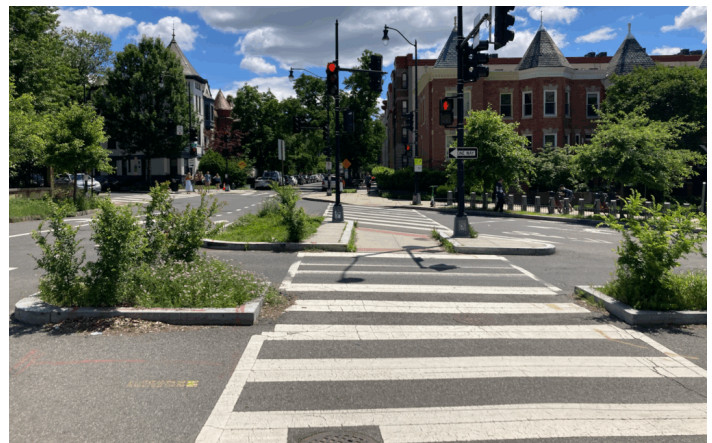
High visibility crosswalk, pedestrian refuge, and curb cuts Source: Smart Growth America
