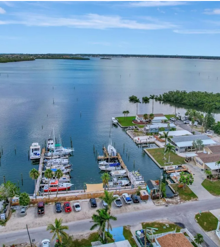
Bradenton, Florida, docks and piers with commercial and residential development Source: Gina Morgando
