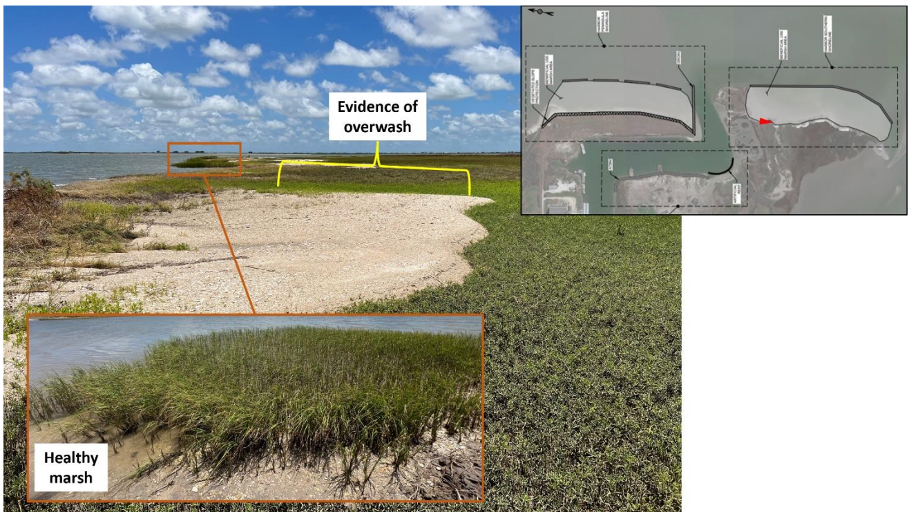
Figure 10. Evidence of overshoot and healthy marsh along the southern shoreline.
