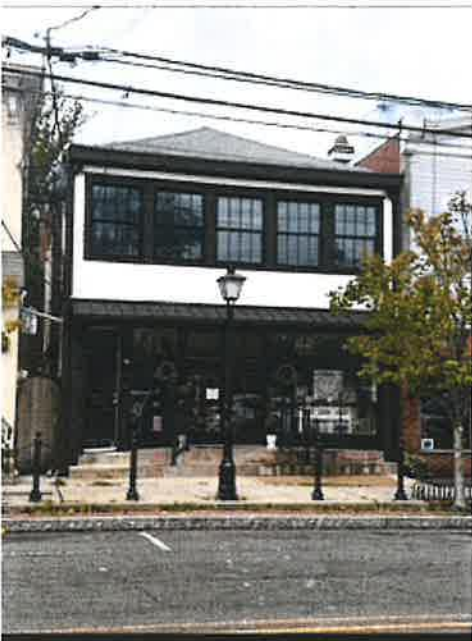
3. New windows + metal awning
