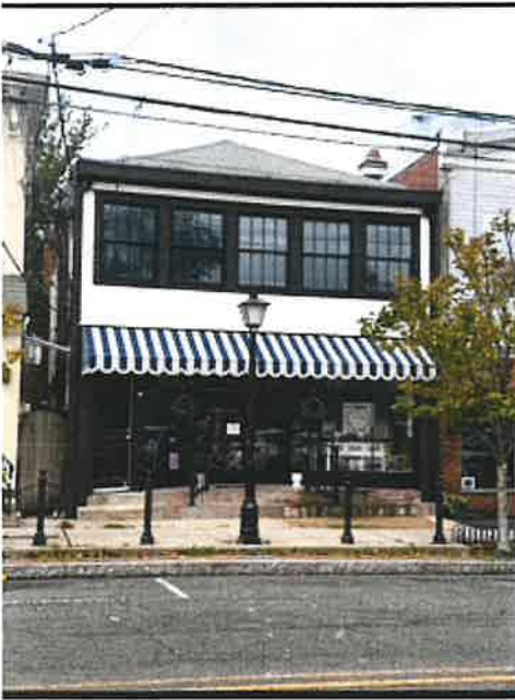
5. New windows + fabric awning
