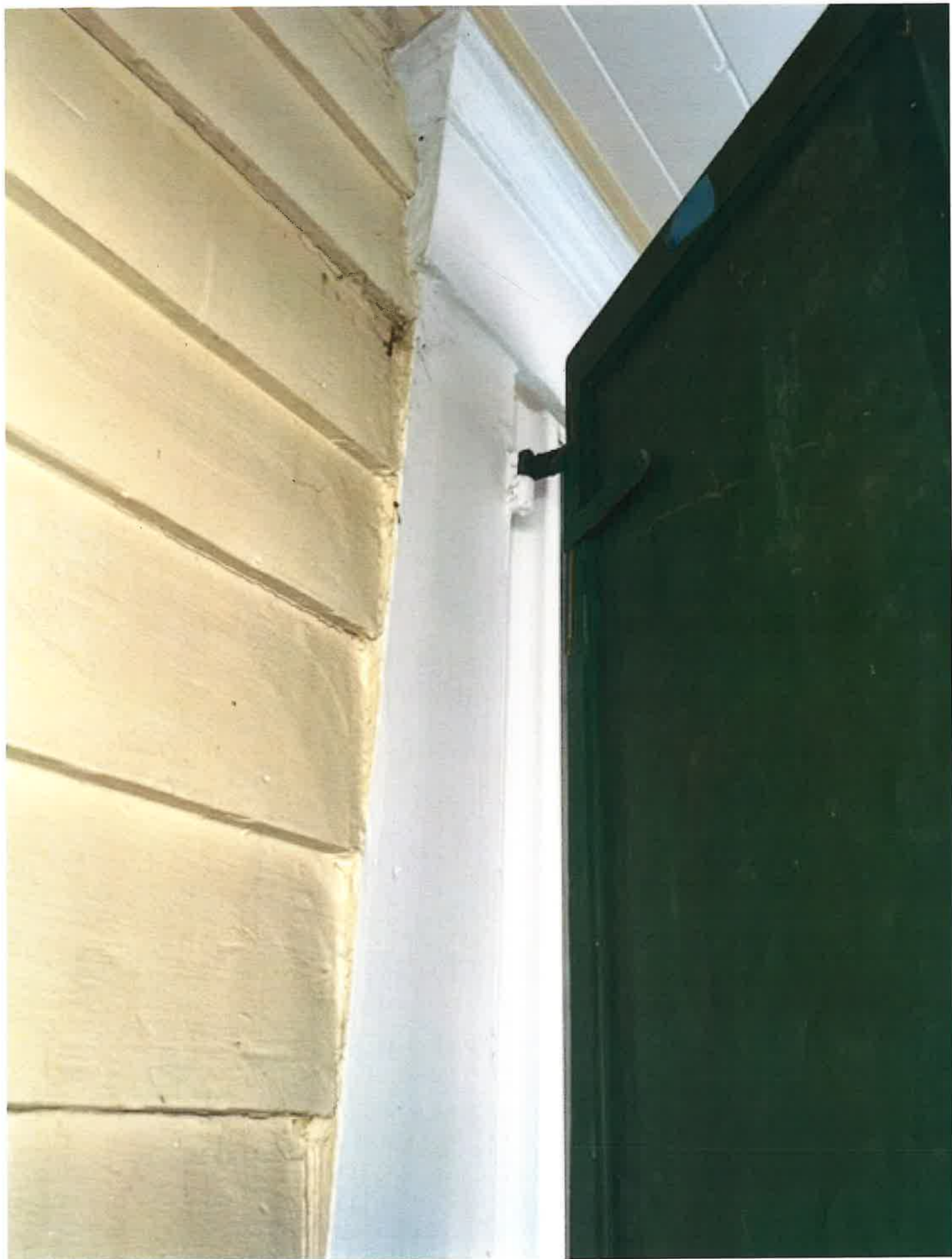
typical street facade window - note header molding
