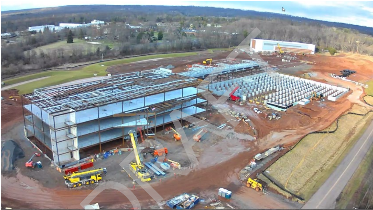
Progress Photo of Building Construction (Foundations for Module Buildings in right portion of photo)
