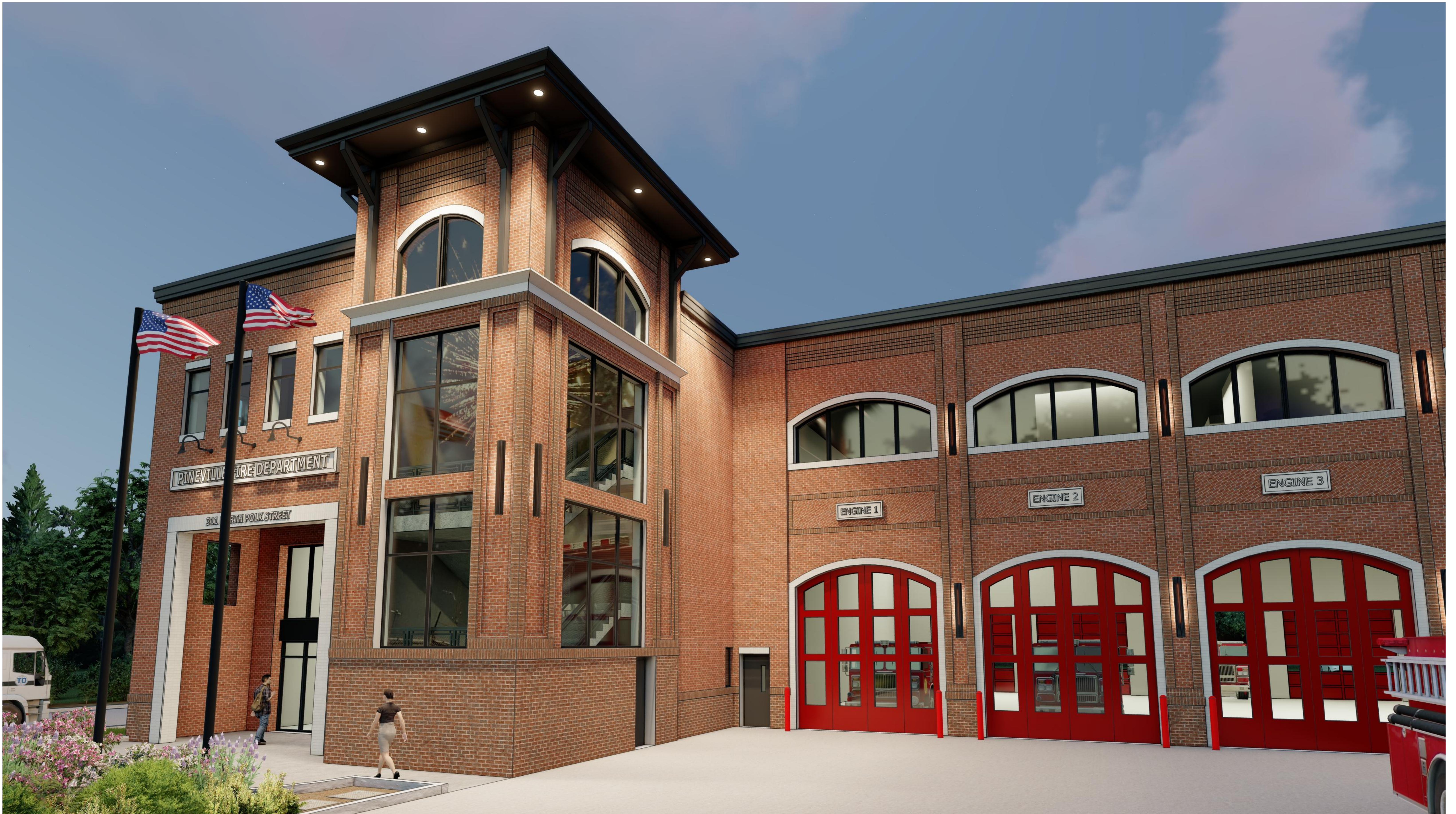
FRONT STAIRTOWER AT DUSK (VIEW FROM FRONT APRON)
