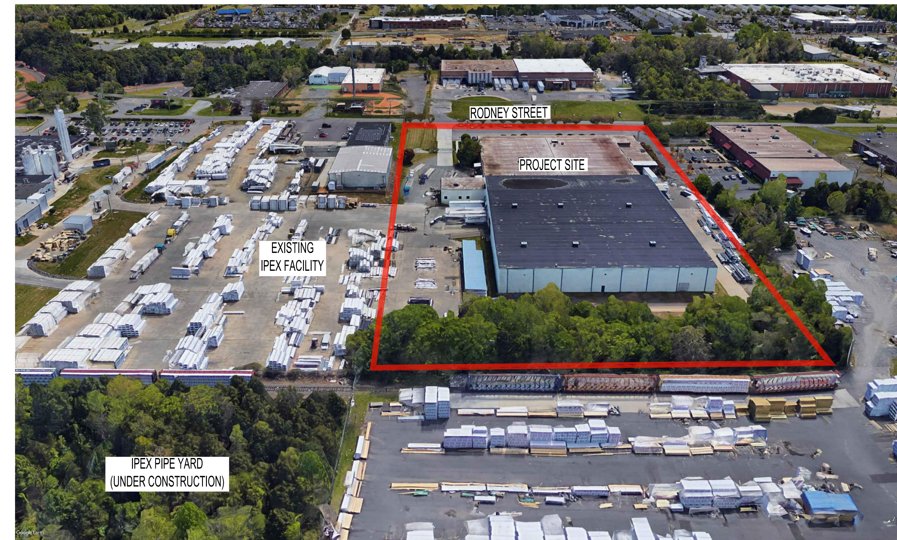
BIRDSEYE LOOKING EAST
