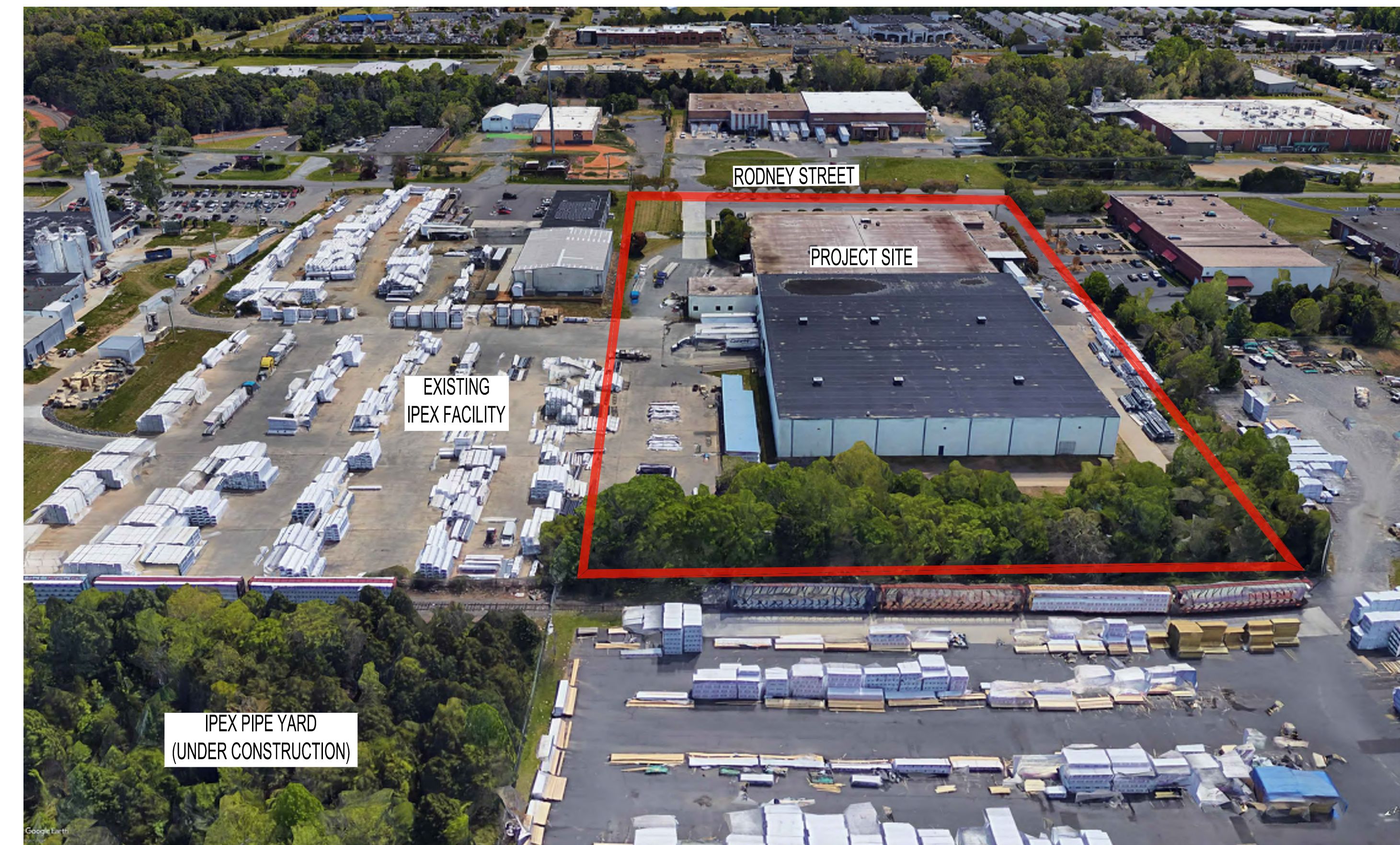
BIRDSEYE LOOKING EAST
