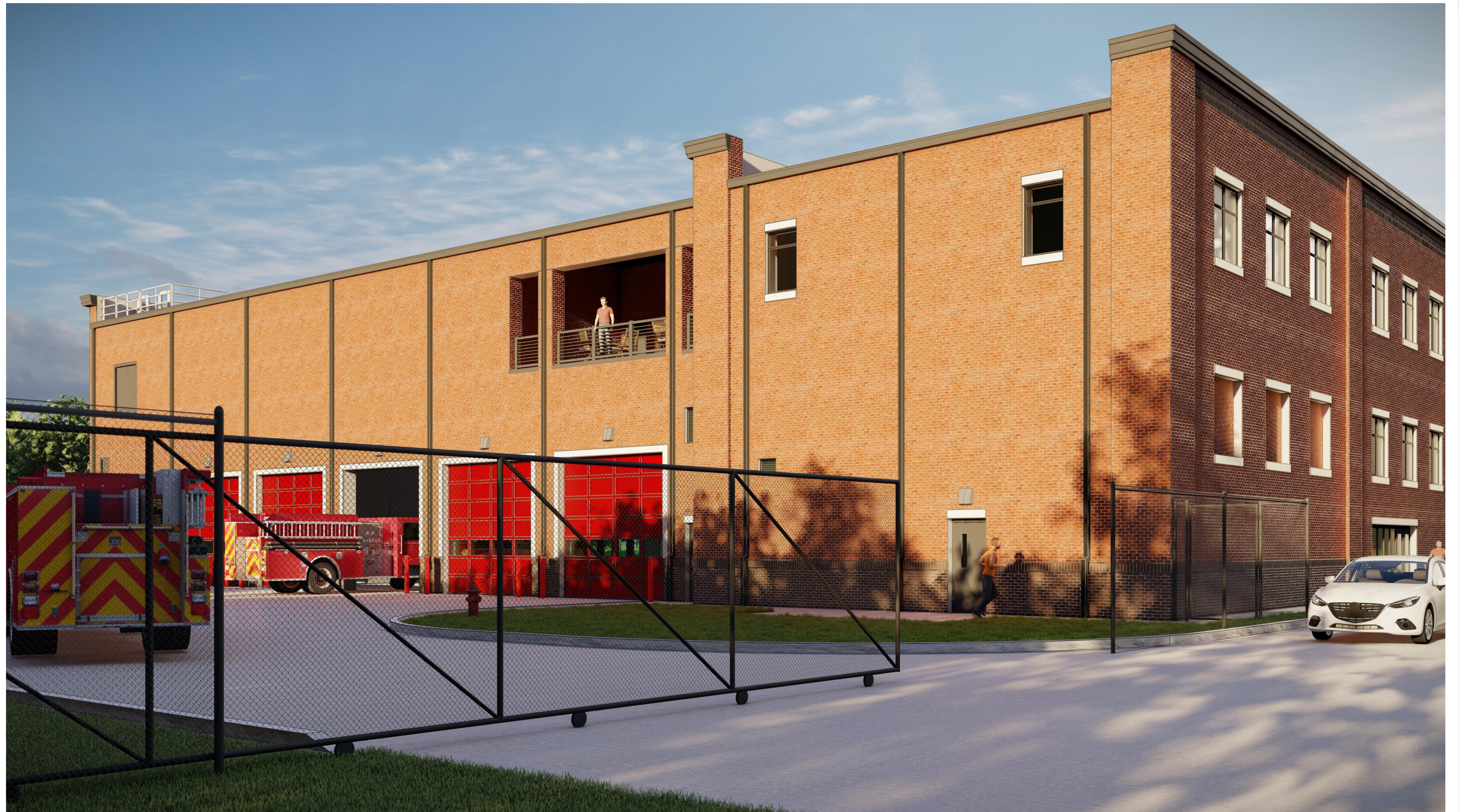
REAR VIEW AT TRAINING ROOM, OUTDOOR PATIO AND APPARATUS BAYS (FROM RETURNING/SHARED DRIVEWAY)
