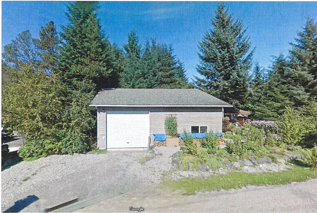
Exterior of existing structure which would be used in its entirety for the school
