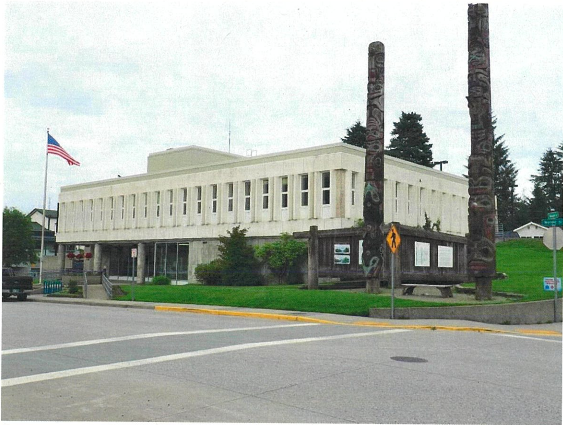
Figure 1. Petersburg Federal Building
