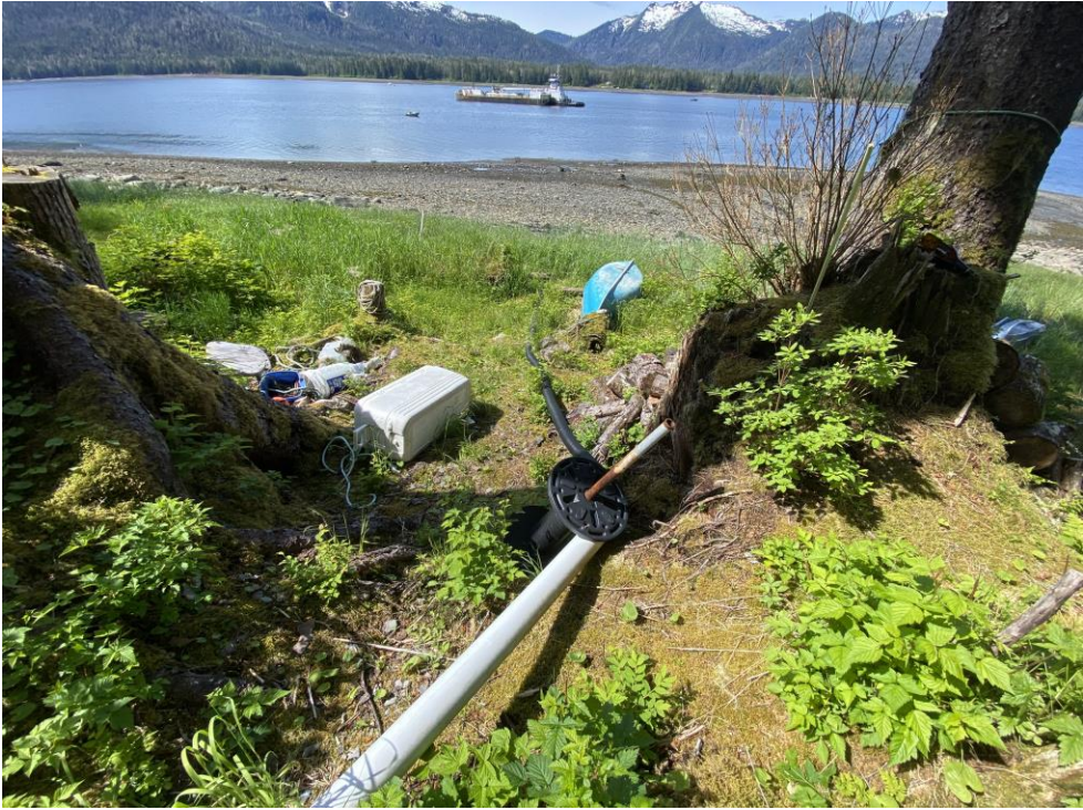
Pipe from septic tank going to beach.
