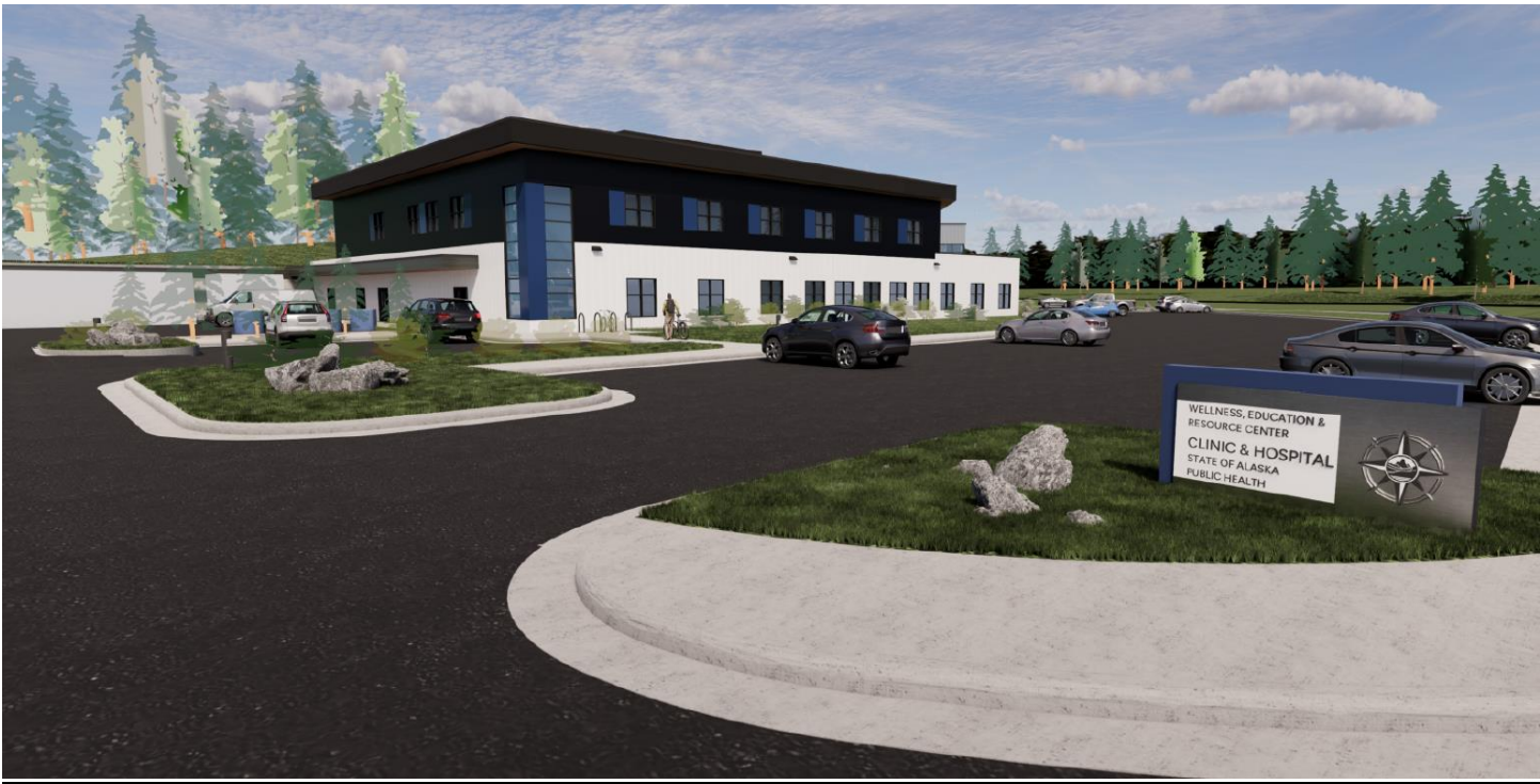
Phase 3 & 4 Completed – Hospital – Looking East from WERC Building Drive
