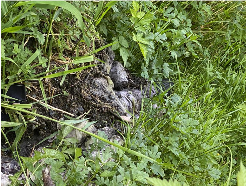
Discharge pipe below house leading to septic tank.
