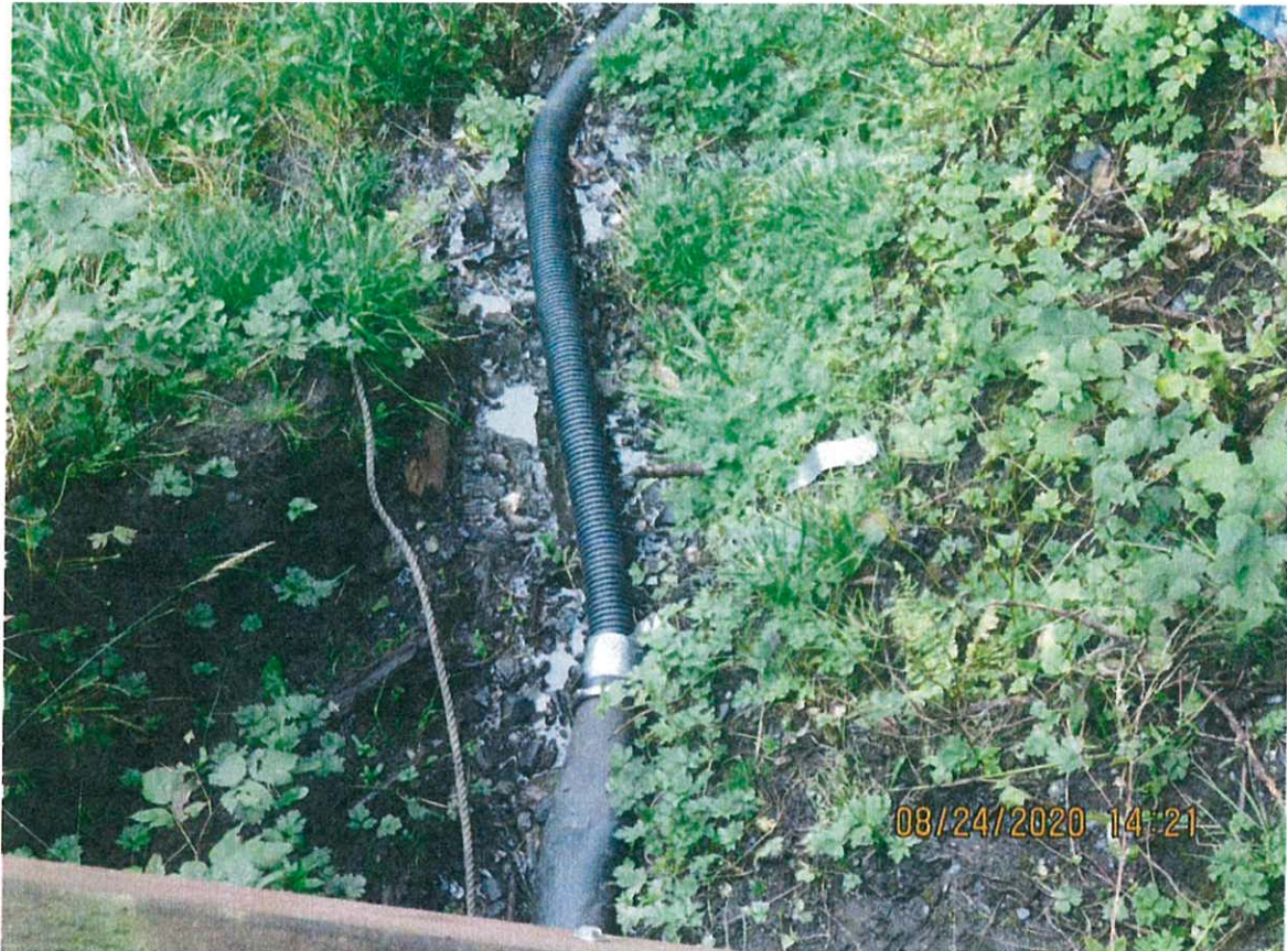
Photo showing connection from original piping to new corrugated drainpipe.
