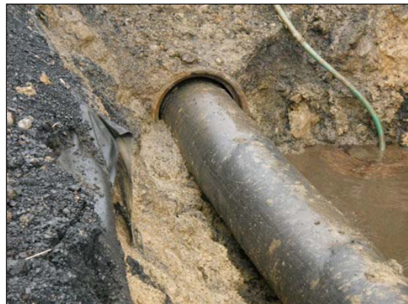
Figure 1: Sliplining with HDPE pipe
