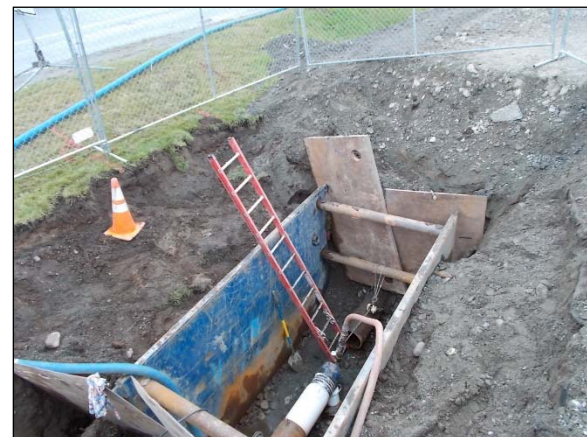
Figure 3: Typical CIPP liner access and insertion pit
