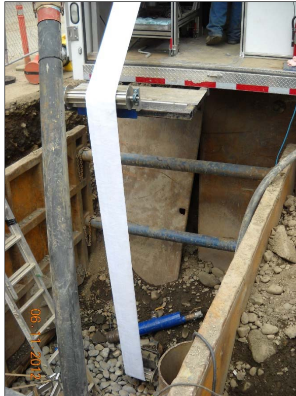
Figure 4: Pull-in insertion of pressure CIPP liner
