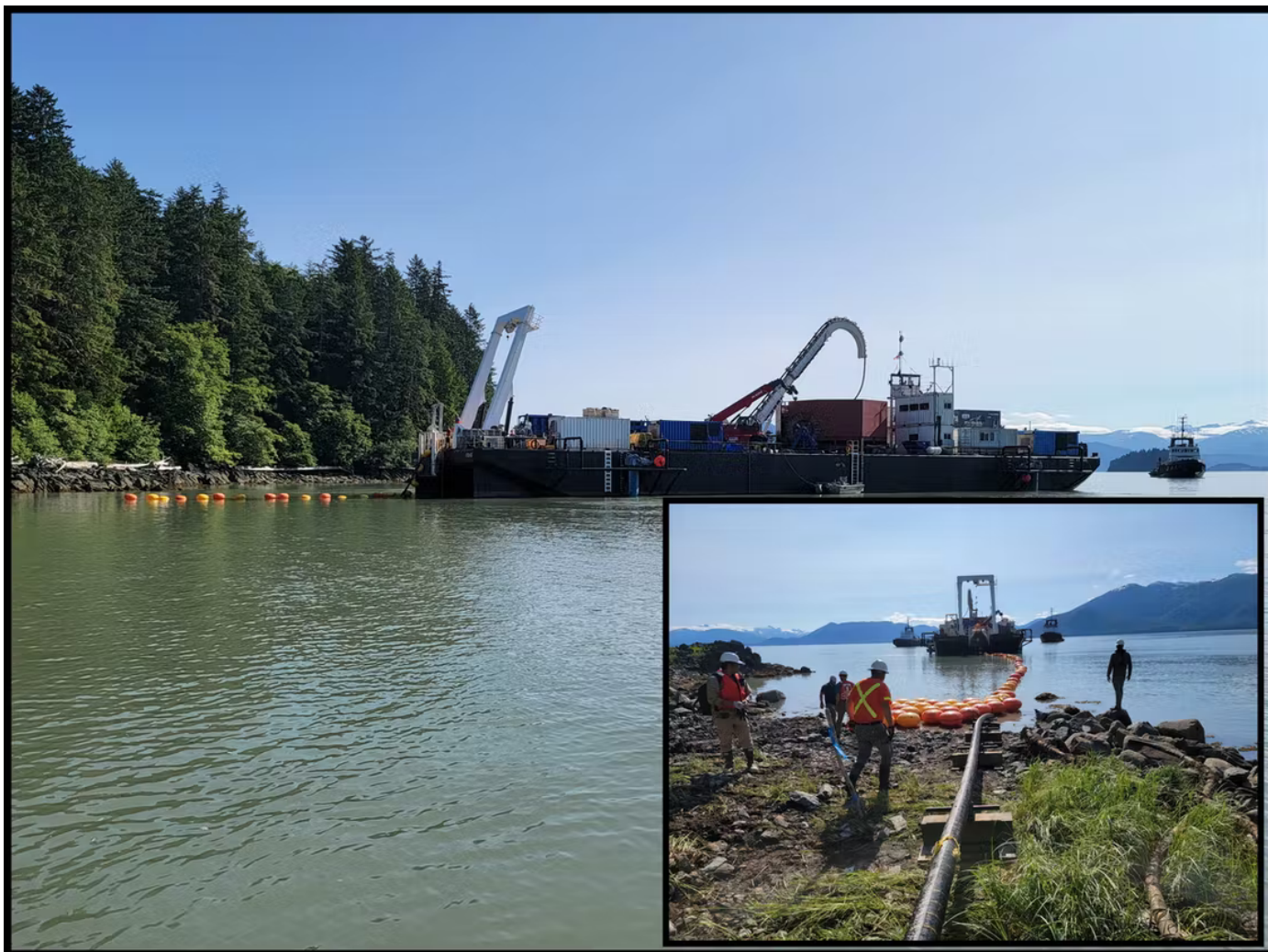
Installation of the 69 kV XLPE insulated cable, Vank Island, Alaska.
