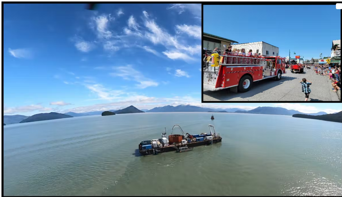
Installation of the 6kV XLPE Insulated cable on July 4, 2021.
