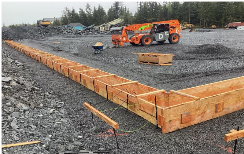
Footing Forms at Grid 1
