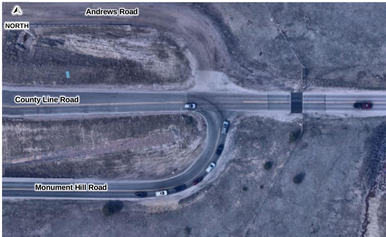
County Line Road & Monument Hill Road
