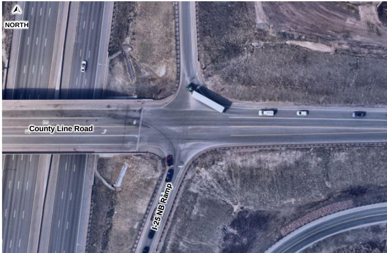
County Line Road & I-25 Northbound Ramp
