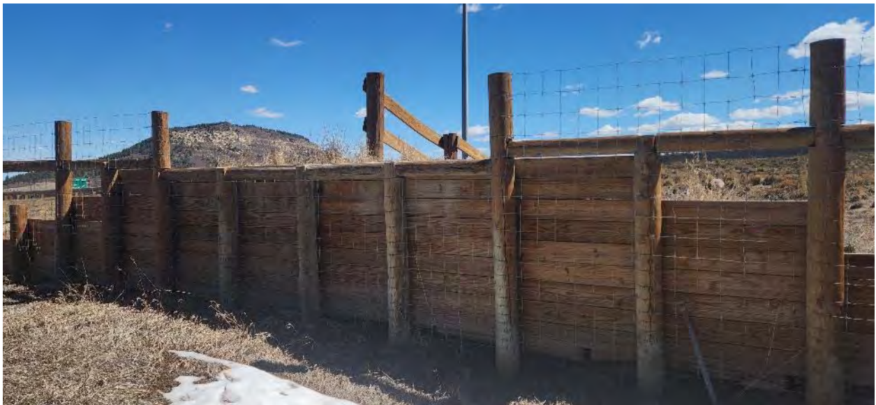
WTP 3: View northeast of wildlife fence and ramp adjacent to I-25.
