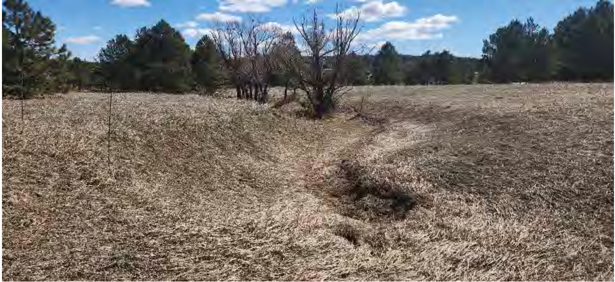
WTP 6: View downstream of Channel 1 near Beacon Lite Road.
