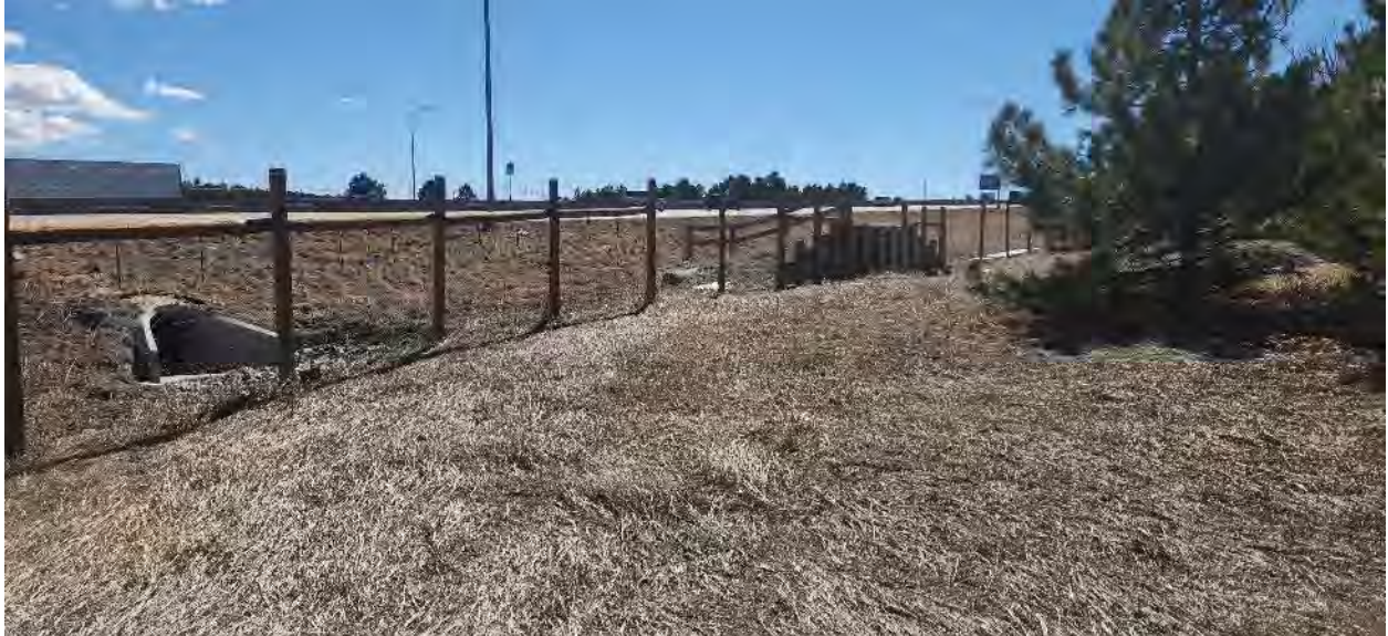
WTP 7: View downstream of confluence of Channel 1, Swale 1 and Swale 2 towards I-25, 24-onche culvert, wildlife fence and ramp.
