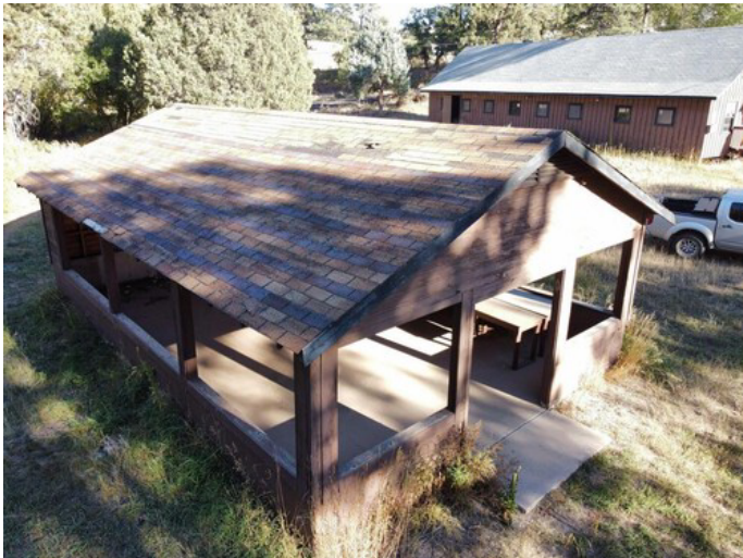
Tear off existing roof system replace with max rib metal system.
