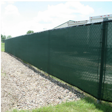
Proposed Fence - 6' weld wire fence w/ screening
