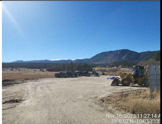
Figure 4. North of property line looking southeast.
