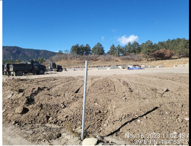
Figure 2. Northeast property corner looking southwest.
