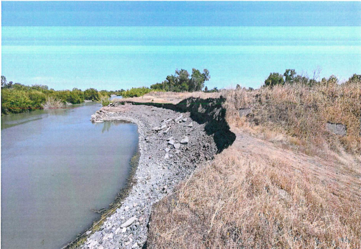
Looking East at the portion of the burn dump that is being impacted by stream flow.
