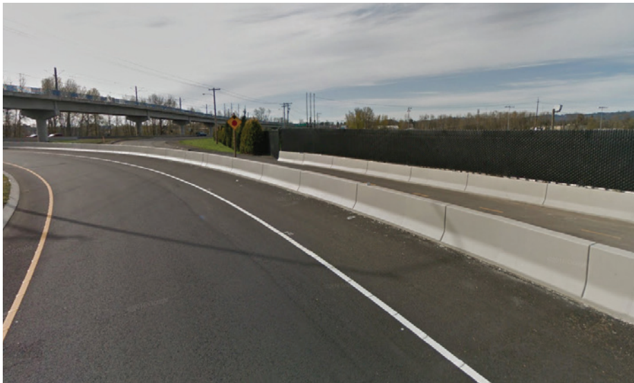
ODOT facility near Portland Expo Center showing protected sidepath w/ shoulder and concrete barrier. A similar facility could potentially be provided along McLoughlin Blvd.
