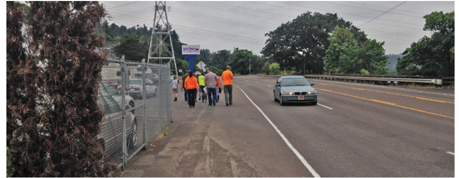
P-1 | McLoughlin Blvd, between S. 2nd and PGE Substation
