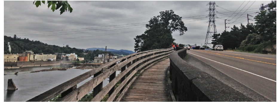
McLoughlin Blvd boardwalk, looking north
