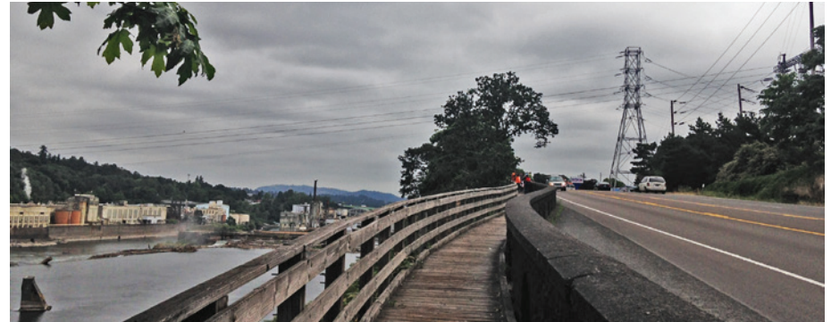
P-1 | McLoughlin Blvd boardwalk, looking north
