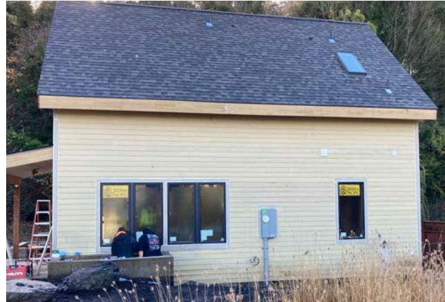
Permitted / As Built
