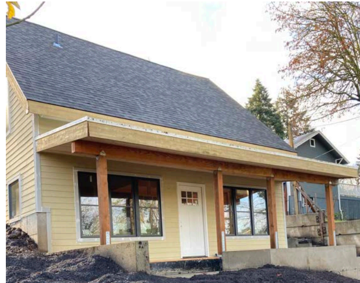
Permitted / As Built
