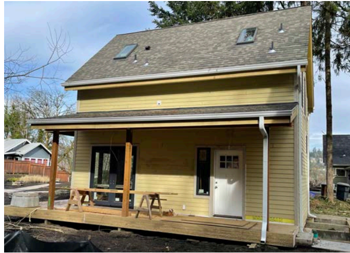
Permitted / As Built
