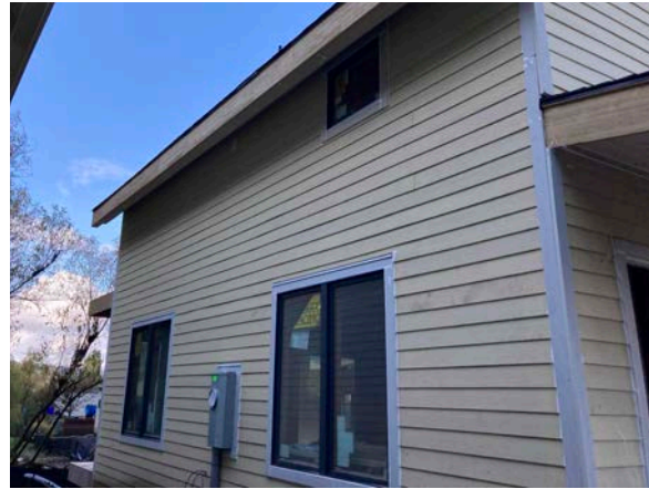
Permitted / As Built
