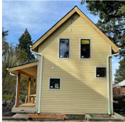
Permitted / As Built
