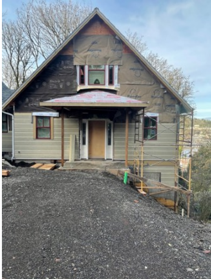
4th Ave New Home
