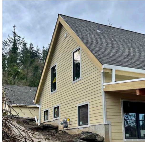
Permitted / As Built
