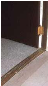
The historic threshold was made accessible with a 1/2" wood bevel. Photo: NPS files.
