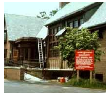
This accessibility ramp is compatible with the historic building in scale and materials. Photo: William Smith.
