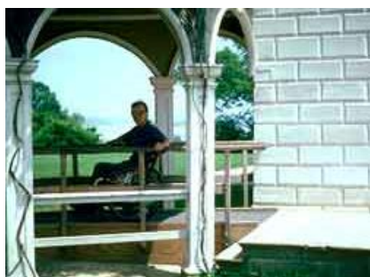
The significant building site is now accessible to people with disabilities (note steps in front of ramp). Photo: NPS files.
