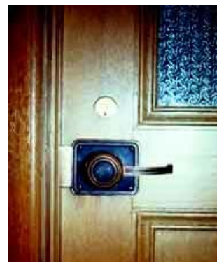
This door handle has been retrofitted to meet ADA requirements. Photo: NPS files.
