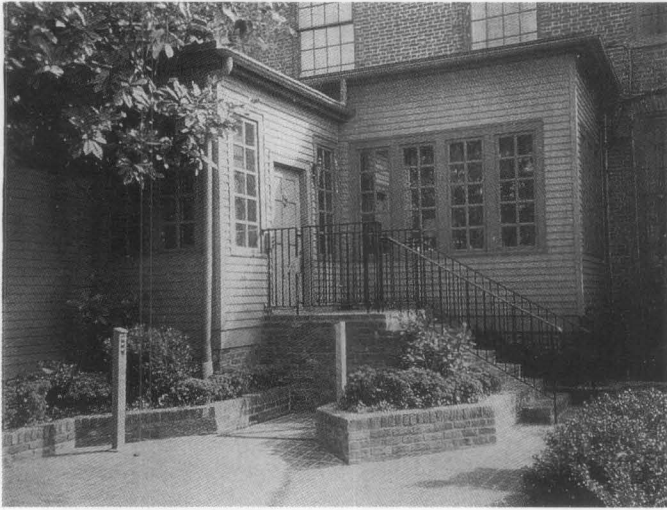
Figure 14. At the Lieutenant Governor's Mansion in Frankfort, Kentucky, a retracting lift (b) was installed to minimize the visual effect on this historic building when not in use (a). Photos: Aging Technology Incorporated.
