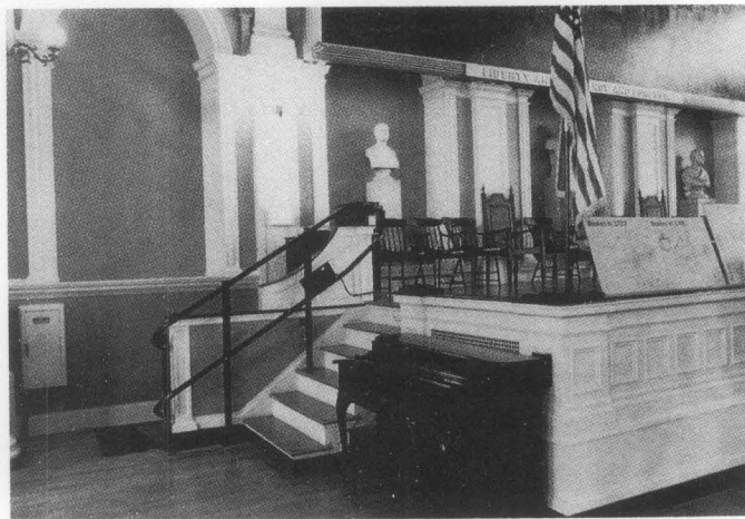
Figure 19. Inclined lifts can sometimes overcome interior changes of elevation where space is limited. This lift in Boston's Faneuil Hall created access to the floor and stage level of the State Room. Photo: Paul Holtz.
