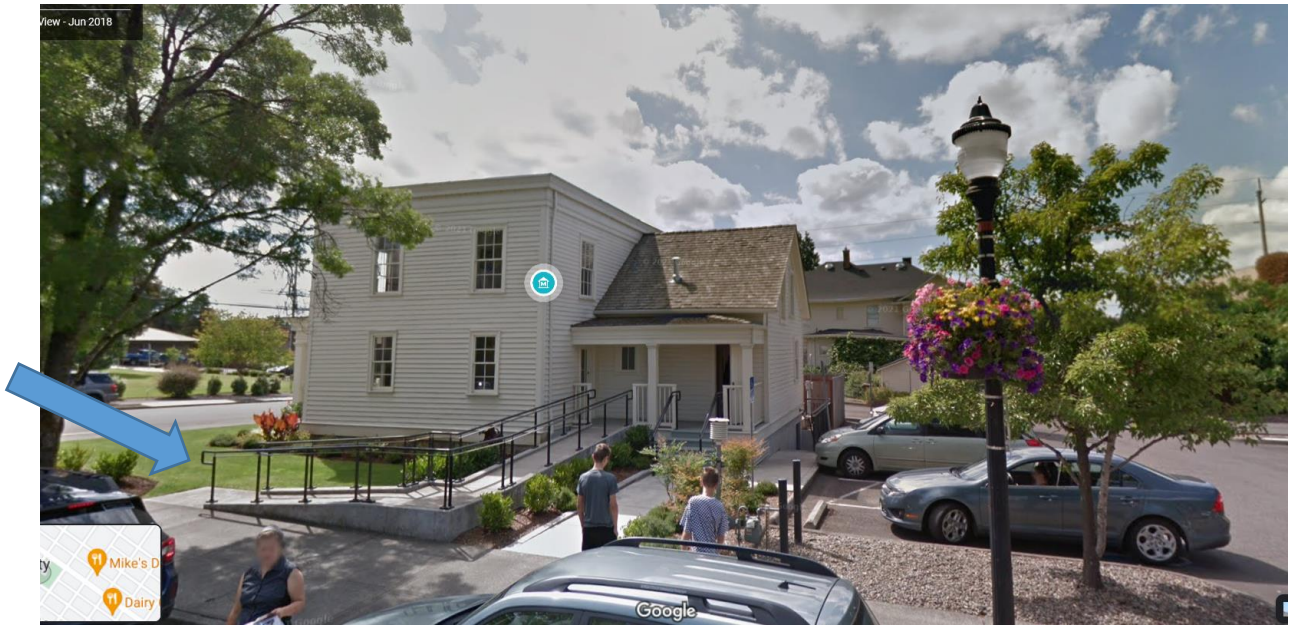
619 6 th Street Ermatinger House ADA ramp (2014)
