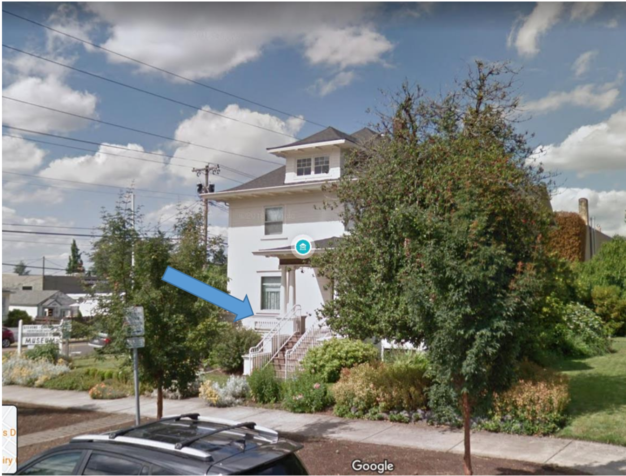
603 6 th Street. Stevens Crawford House metal hand railings (2009)
