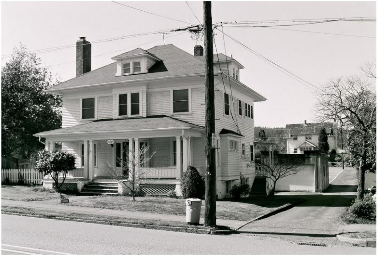
Figure 8 -909 Washington Street- Charles Caufield House. An example of a side porch and stair with a 3 ½ to 4-foot foundation height on a sloping site.
