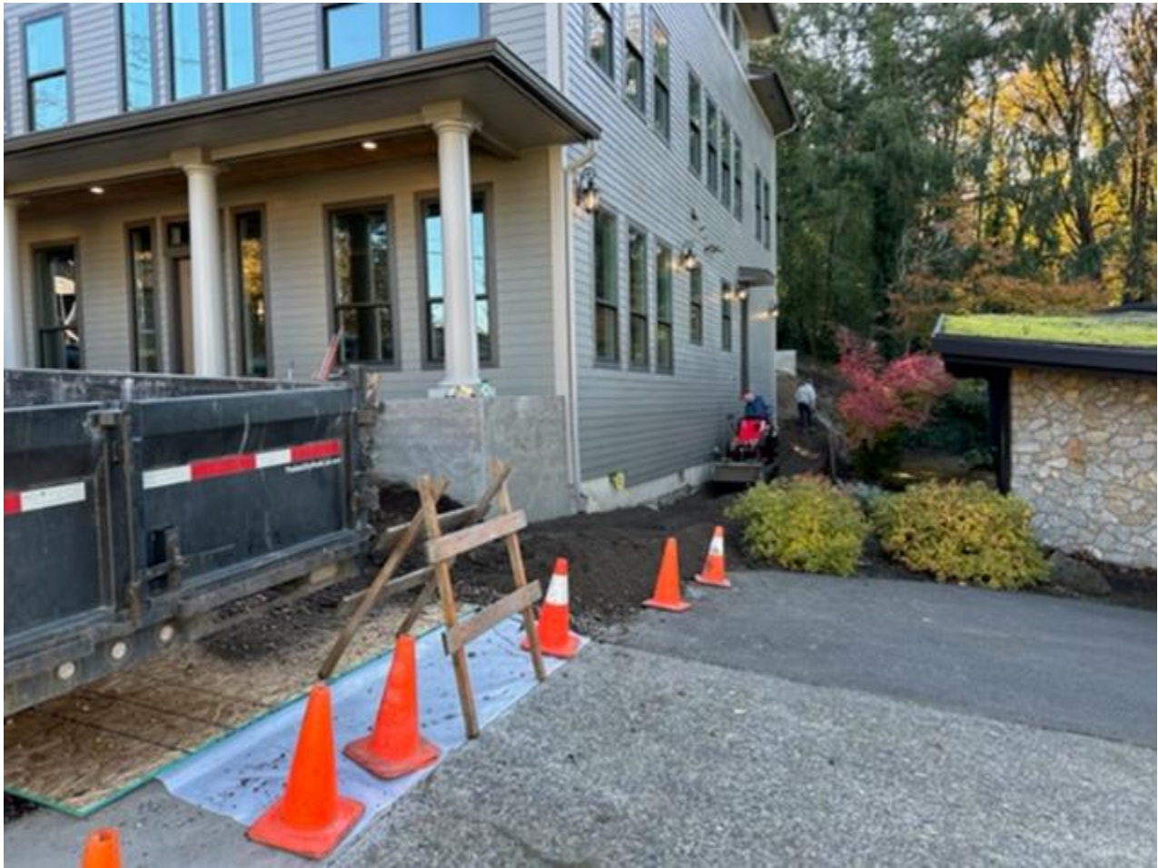
Figure 5 existing condition, photo taken November 17, 2022. Note unpermitted CMU wall is removed.
