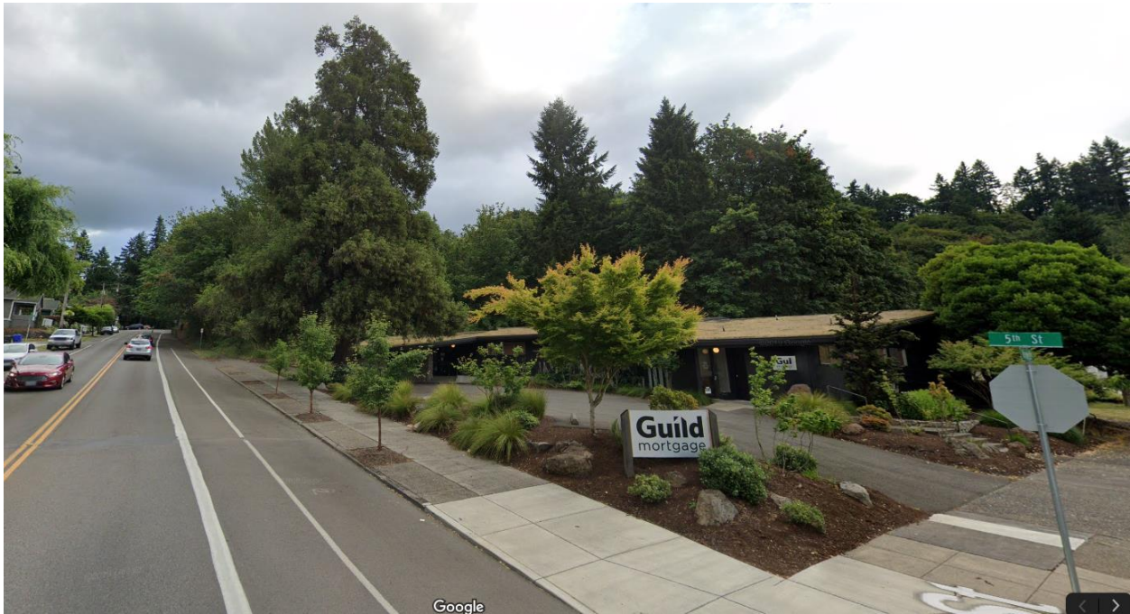
Figure 6 Neighboring building at 1010 5 th Street; a modern commercial building with a low shed roof, roughly U-shaped. The offices are sited in the eastern portion of the building, with a small courtyard framed by the low roof on the west side. The building is primarily clad with stone veneer, but some portions have vertical groove plywood siding. The windows are fixed aluminum sash and are located primarily on the east and west sides of the building. It is not a designated structure in the Mcloughlin Conservation District. (Google Maps- taken prior to construction)
