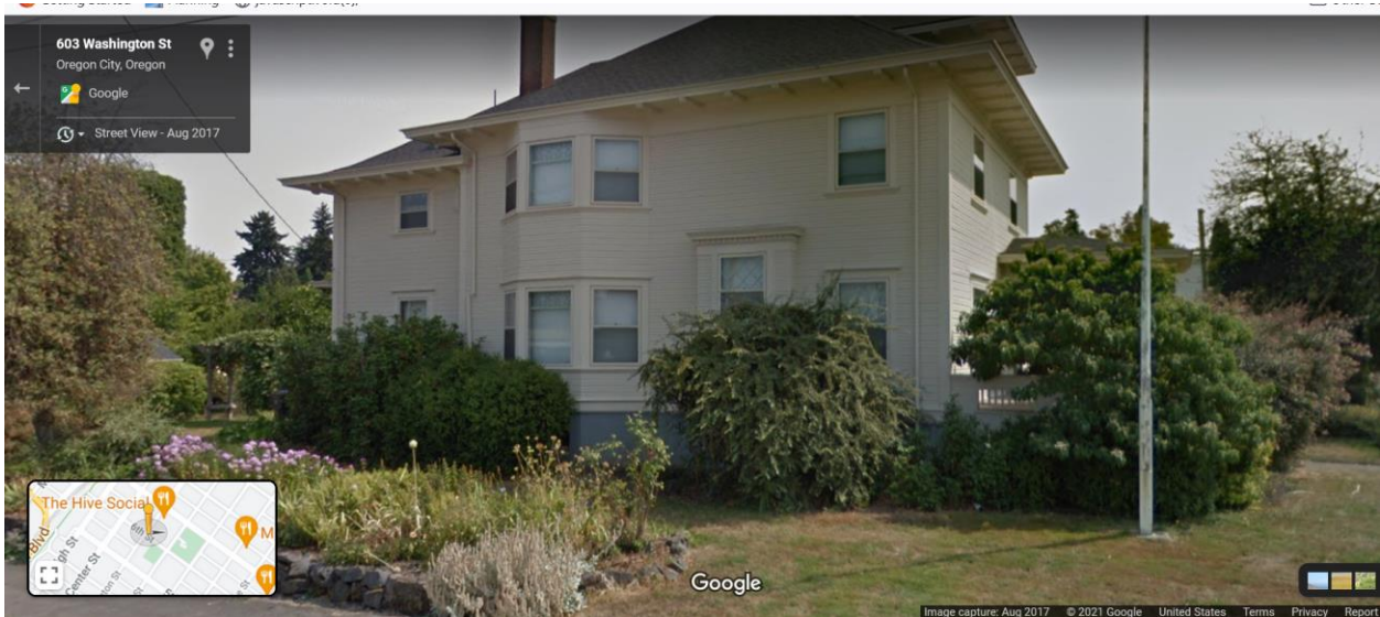
Figure 7-Stevens Crawford House, 603 6 th Street. An example of a larger Foursquare/bungalow design with a foundation height of 3 ½ to 4 feet.
