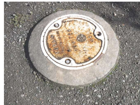
Photo 5-F: Flush Mount Monument for Groundwater Samples Monitoring Well Along Gravel Access Road Right-of Way.
