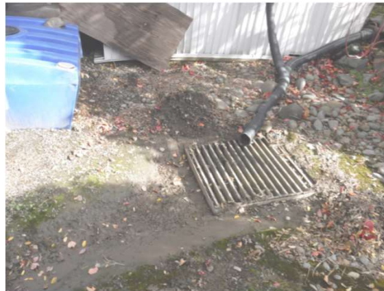
Photo 3-E: SW Catch Basin and Septic Holding Tank (blue).
