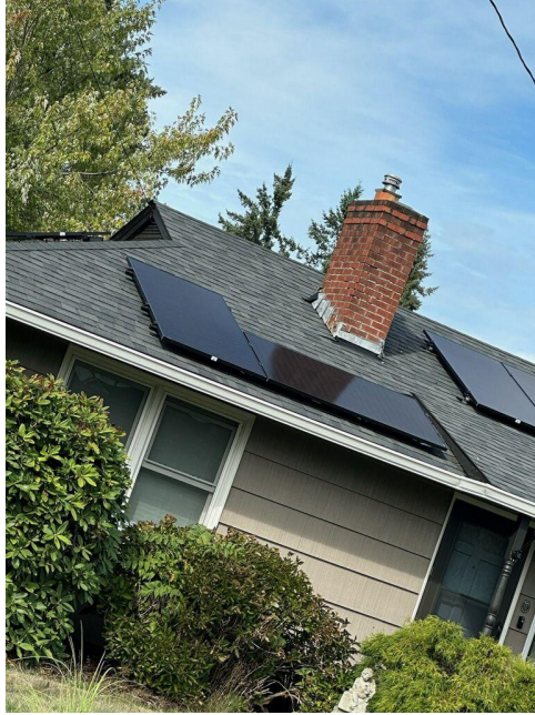
Panels installed on Beverly Dr.
