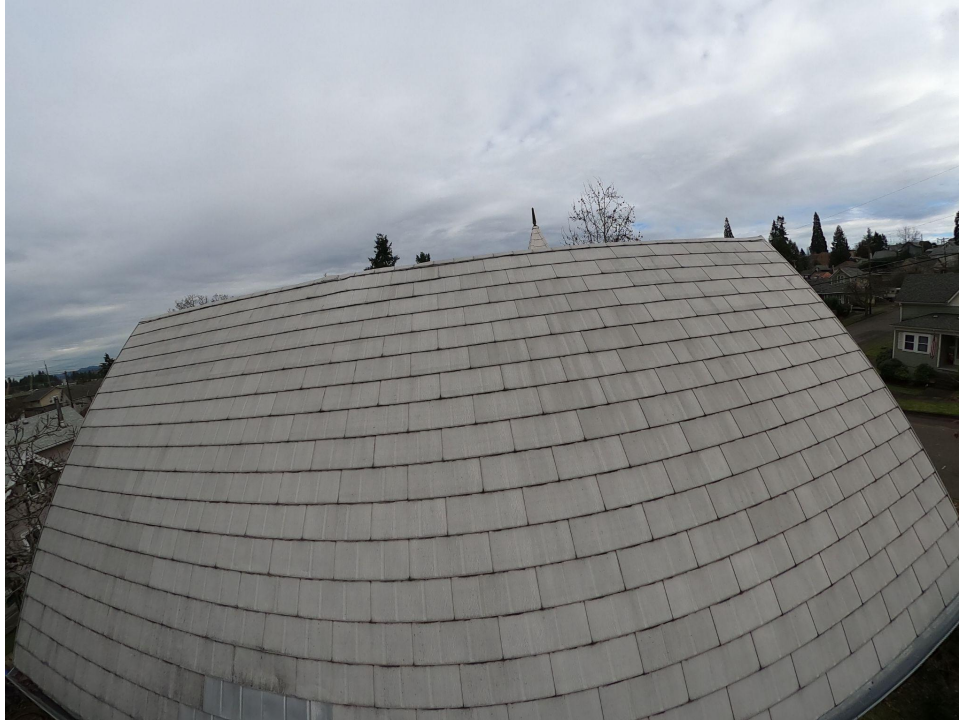
Back Roof Section - 7 panels will be installed on this roof section.
