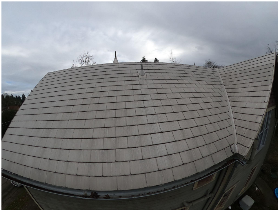
Right Roof Section - 2 panels will be installed on this roof section.
