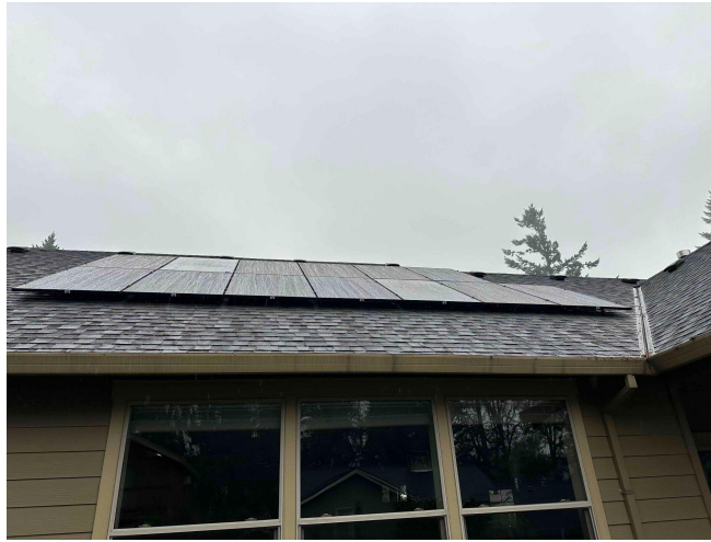
Panels installed on Charman St.
