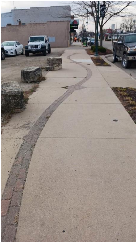
Paver band and diamond settling
