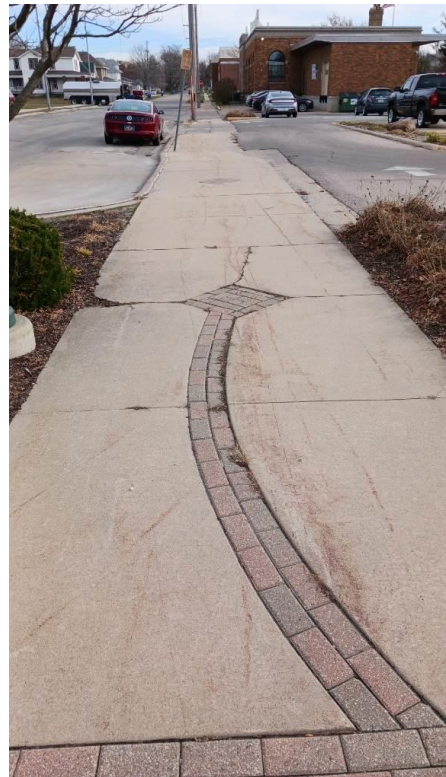
Paver and diamond settling
