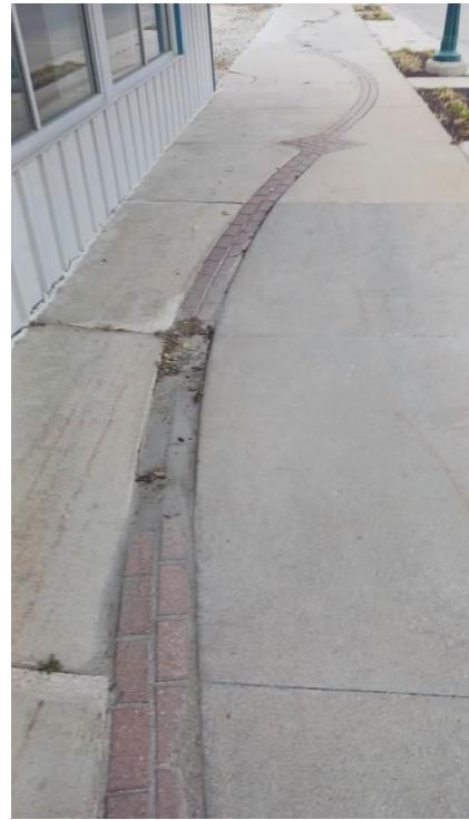
Paver band setting greater than 0.25
