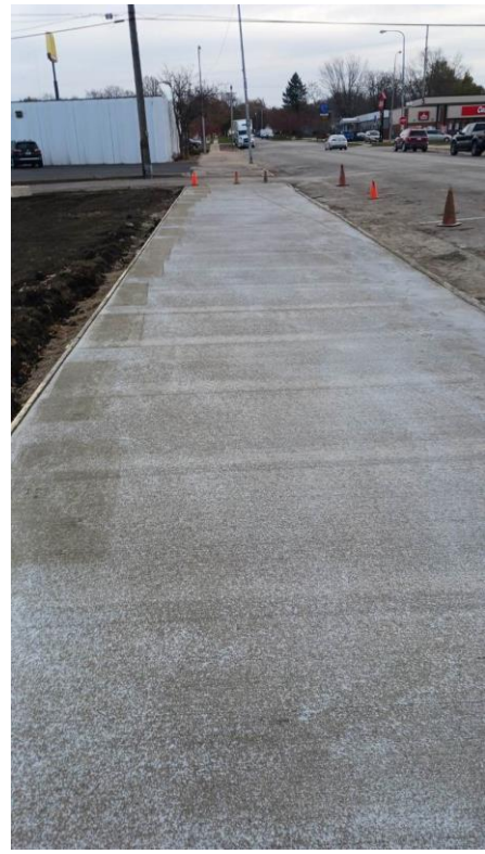
New sidewalk with greater than 2% cross slope
